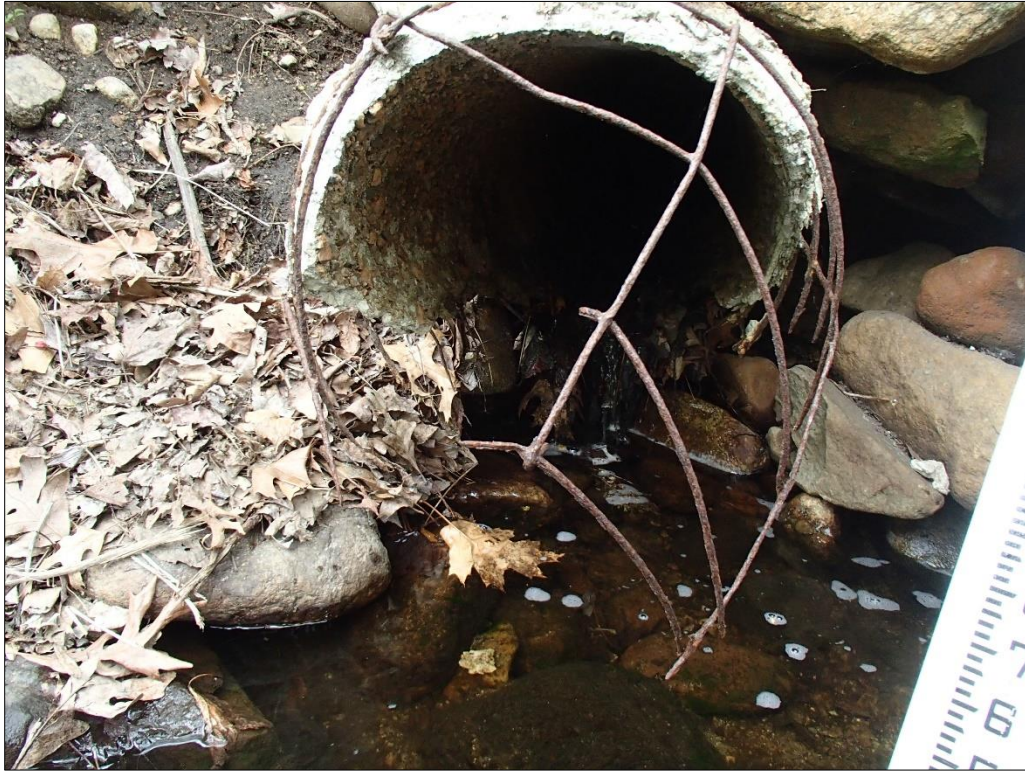
Photo 5 Looking East: Secondary Pipe Deteriorated
