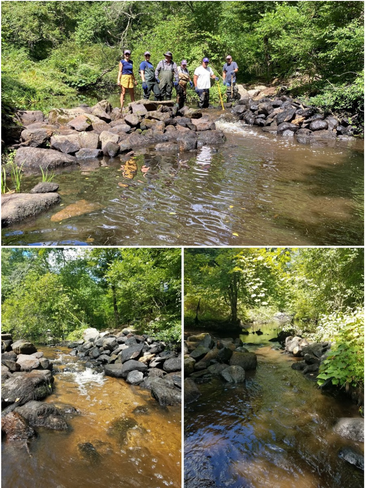
Figure 18. Low flow channels created (above) to improve passage at the upper weir (left) and lower weir (right) at the Whelden Cotton Mill (WCM) by DMF staff (August 31, 2022).
