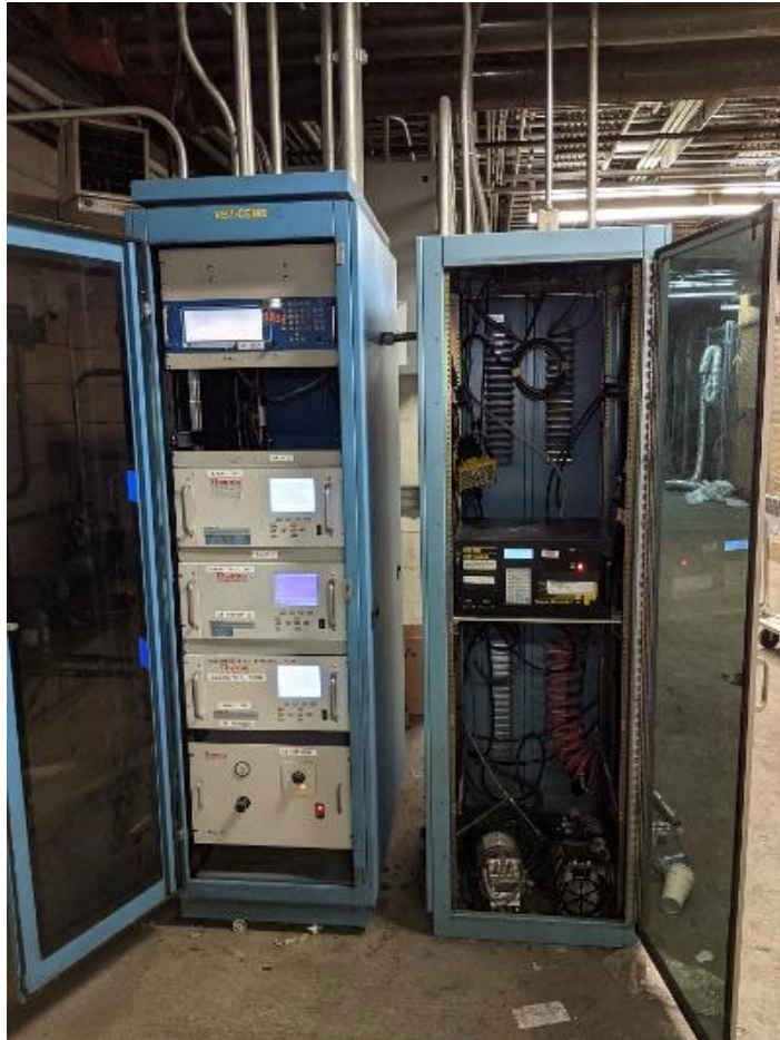
FIGURE 3-3: CO MONITORS LONGITUDINALLY FOR VENTILATED TUNNELS
