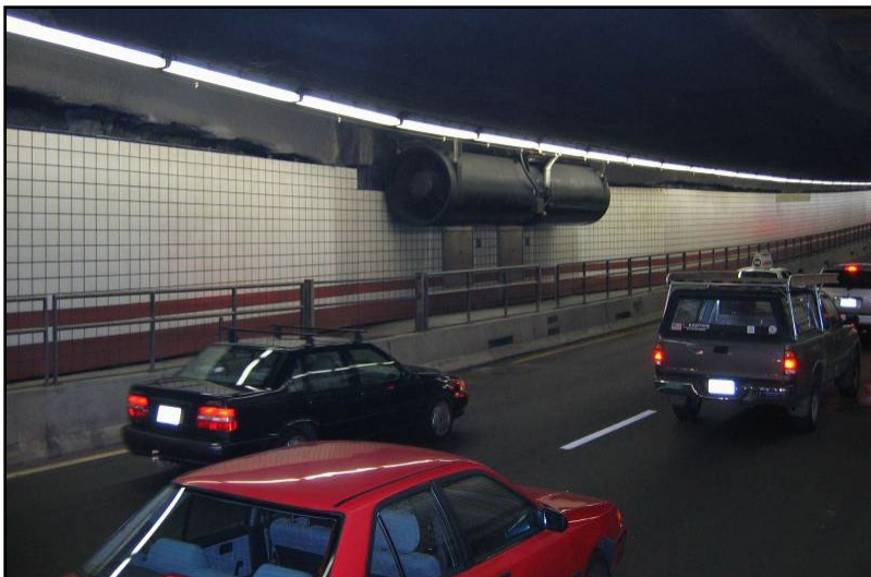
FIGURE 1-16: JET FAN AT LONGITUDINALLY VENTILATION RAMP
