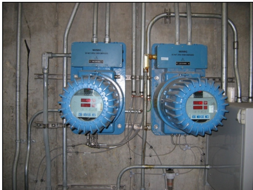
FIGURE 3-3: CO MONITORS LONGITUDINALLY FOR VENTILATED TUNNELS
