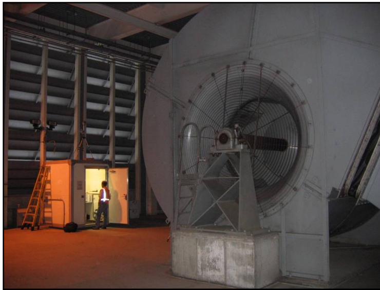
FIGURE 1-15: SUPPLY FAN AT VB 7 AIR INTAKE FLOOR
