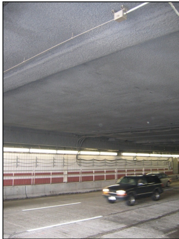
FIGURE 3-1: CO CEILING MONITORING PROBE AT DST
