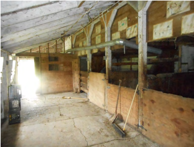
10. Posts in the rear shed between stalls support a roof purlin.
