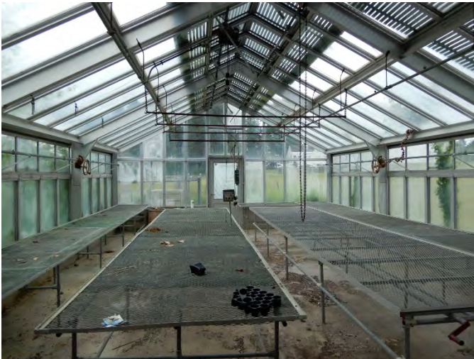
5. Green House wing framed with extruded aluminum shapes using rigid frame design. The knees have brackets to form rigid joints. The aluminum structure is supported on a concrete knee wall.
