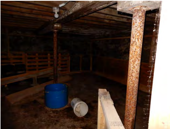
10. View of steel pipe columns showing a rust scale.
