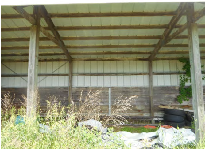
3. Front view of typical bay framing. Front and rear posts support a truss frame. The top chord, a 2x12, supports 2x6 rafters spaced at 24 inches.
