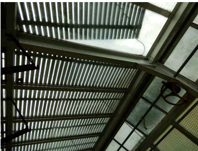
6. View of one half of an arch ridged frame. The rigid frames carry roof purlins and wall girts. Glazed panels in sash and rafter mullions complete the construction.
