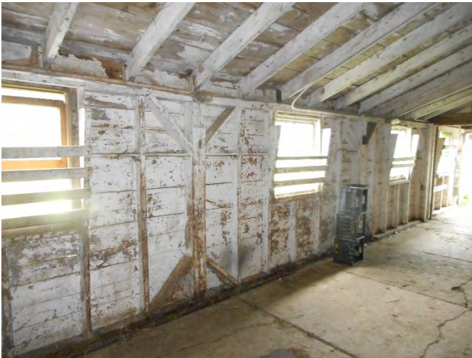
11. The rear wall is wood stud framed supporting dimensioned lumber rafters.
