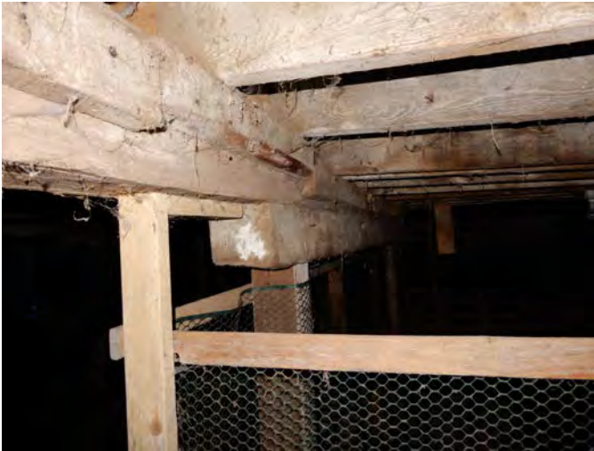
9. View of reinforcement under beam at first floor. The reinforcement is not consistent throughout the floor.
