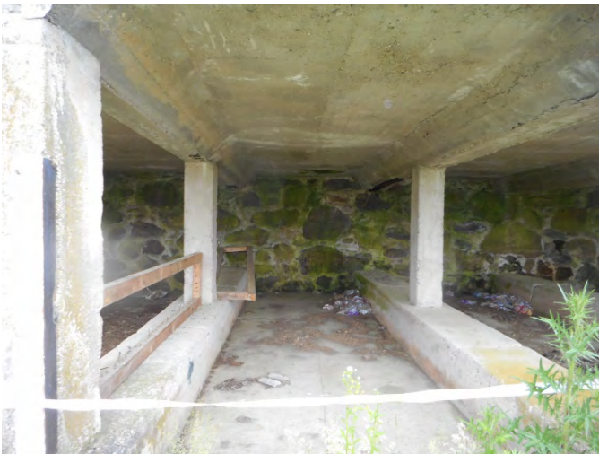
6. Typical stall bay at lower level. Concrete piers support steel beam encased in concrete which in turn supports a one way concrete slab.
