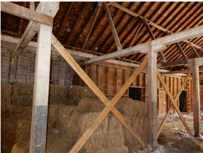
3. Roof purlin in the background propped on the eave tie beam.
