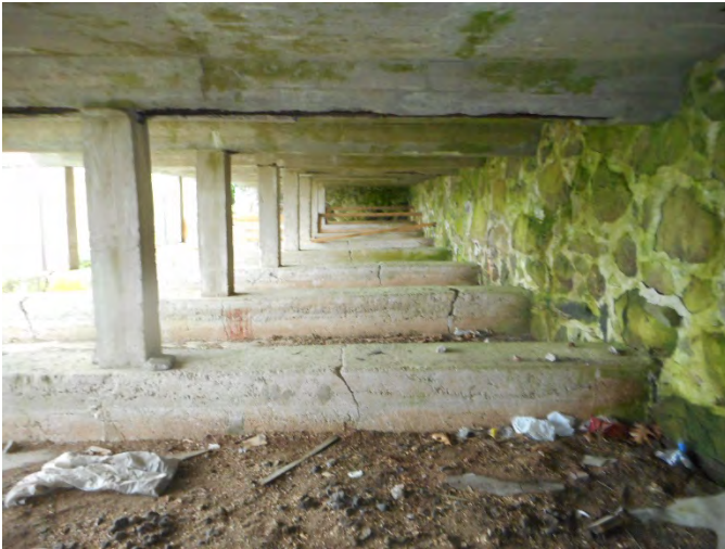
10. Multiple bays viewed down inner rows of piers and foundation wall. Some sleepers are cracked.
