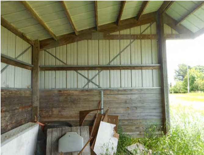
4. Interior view of end wall framing.
