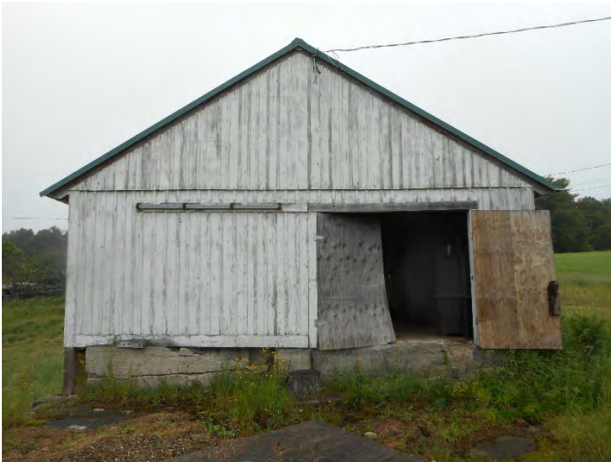
4. End wall to left of front. Left half of foundation wall is cracked and spalled. The upper portion of the wall is wood framed.
