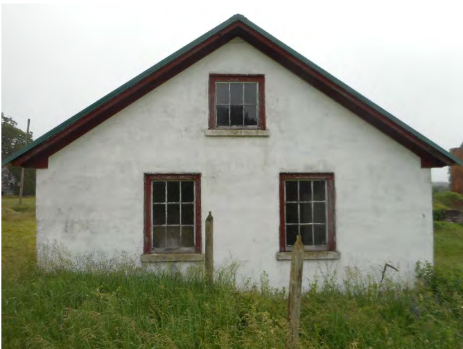
3. End wall to right of front. This end wall is made of concrete.
