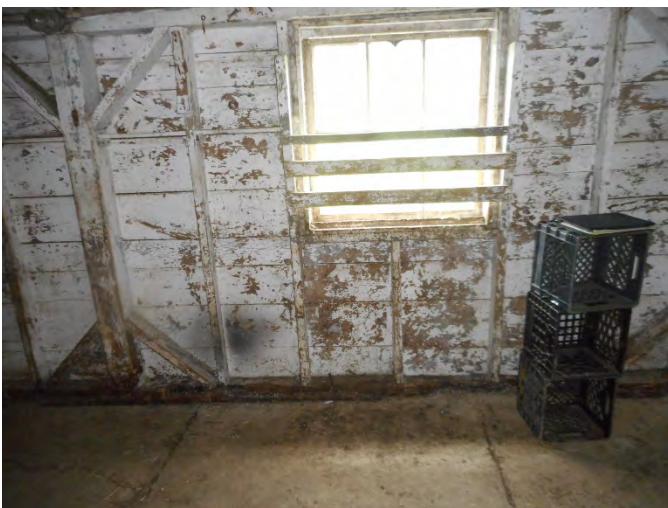
12. The sill of the rear wall is rotted in some locations.
