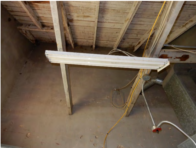
2. Rafters supported on exterior wall at eave and central wall along ridge. Tie joists serve to support hung ceiling tile.
