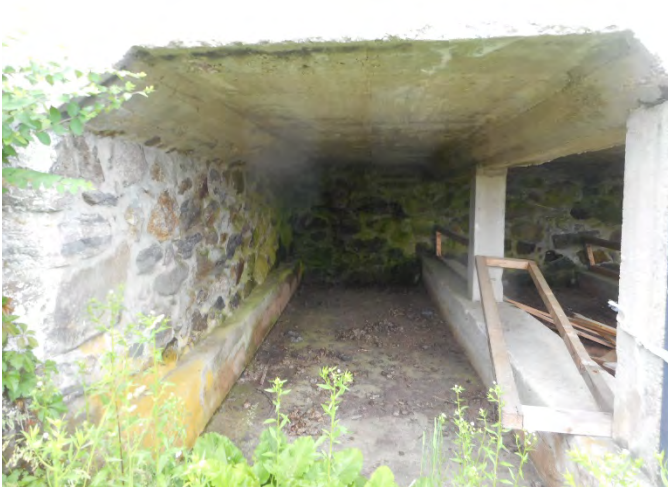
5. End bay of lower level stall. Foundation is rubble stone. Support sleeper and piers are concrete.
