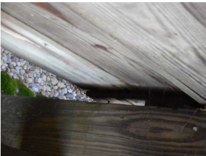
6. View of sheathing along the ground (photo is rotated 90° clockwise) is pulled away from the post likely the result of equipment bumping into the wall.
