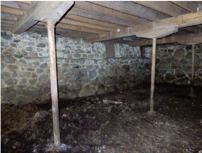
5. Posts supporting the first floor beams are immersed in wet soil that contains urine.
