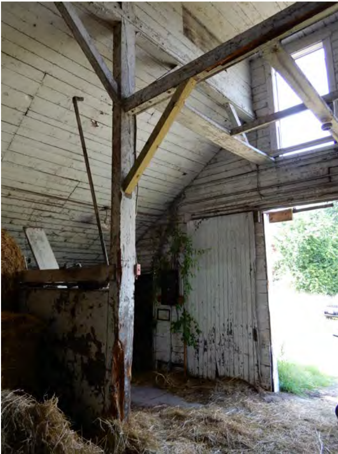
8. Closer view of door opening. Monitor frames into end wall. Post framing in line with the monitor wall is missing inside the end wall. Knee braces here serve to shorten column unbraced lengths and are needed.
