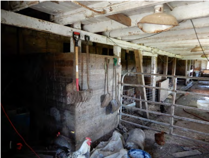
4. Lower shed space. Note in the background the large space between posts supporting the loft beam.
