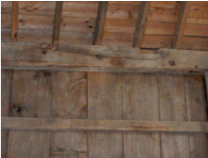
7. View of eave framing at interior of main barn.
