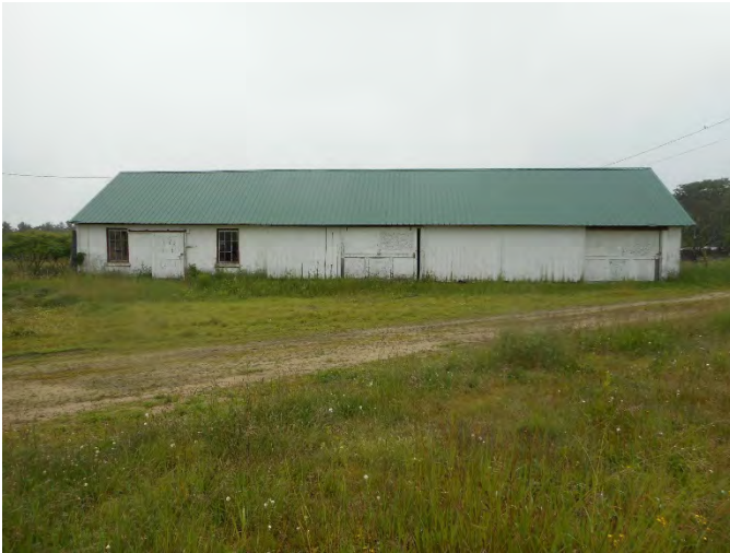
1. Front of Old Cow Barn viewed from access road. Portions of the wall are concrete, and others are wood stud walls.
