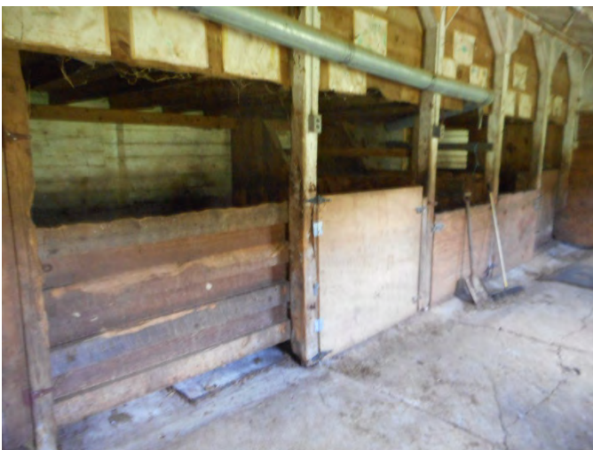
9. Posts between stalls in the rear shed are closely spaced.
