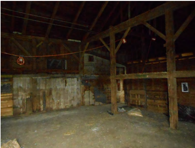
8. Some walls are covered on the interior side of framing as well as on the exterior concealing structure.
