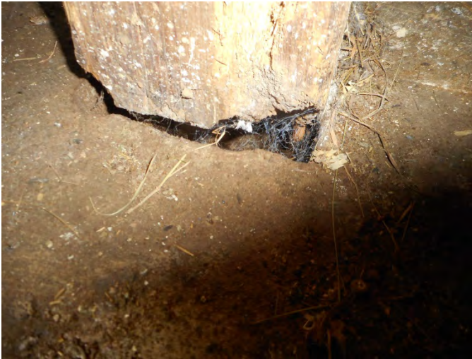
7. Close up view of interior column showing gap under post.
