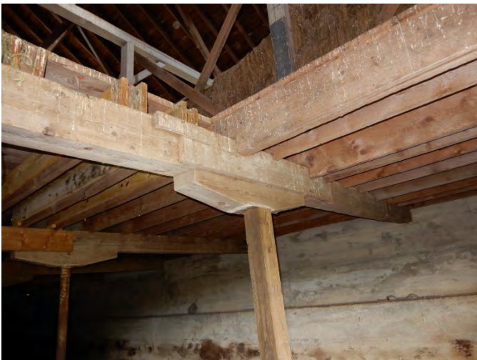
6. Post in upper background that supports the roof purlins is on the first floor beam and offset about two and one half feet from the lower post supporting the floor beam.
