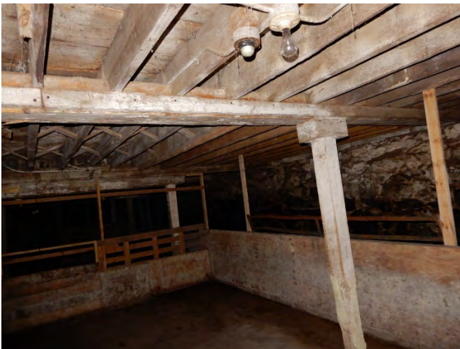
8. View of the underside of first floor framing in the main barn.
