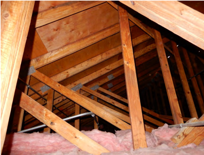
4. Roof framing viewed from hole in ceiling. There are prefabricated wood trusses with metal tie plates. The roof is sheathed with plywood.
