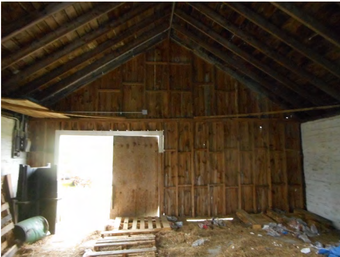
14. Upper end wall over shore stall below. This is a wood stud wall.
