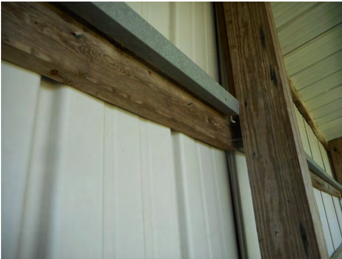
5. Wall girt pulled away from post likely the result of equipment bumping into the wall.
