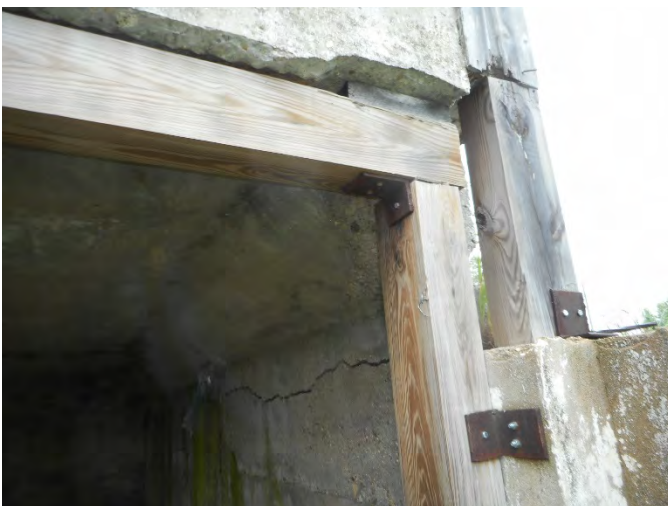
12. Another view of the shoring at the other end. This end foundation wall is made of concrete.
