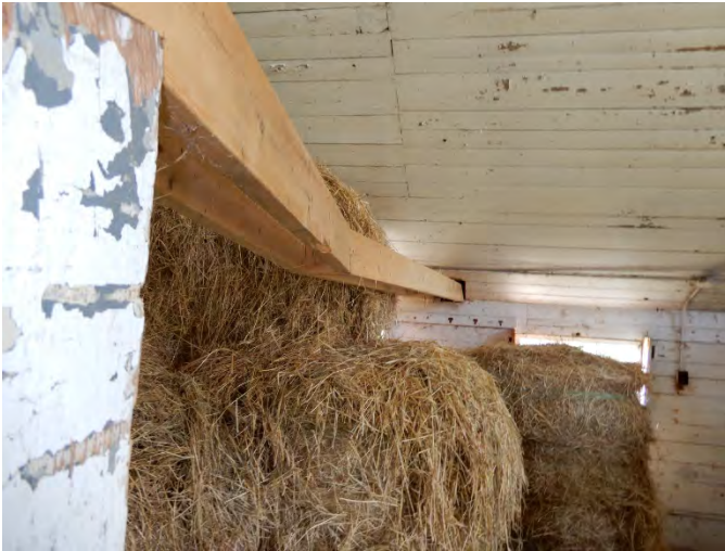
7. Replacement 6-2x6 eave tie broken by equipment moving hay bales.
