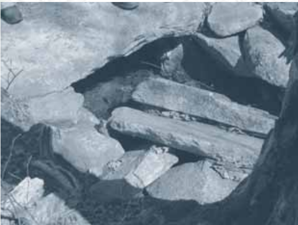
One of the two slabs from this crossing has broken and collapsed into the stream below.
