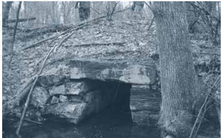
The substantial amount of soil and vegetation on this still-functioning masonry culvert is testament to the skill of the builder.
