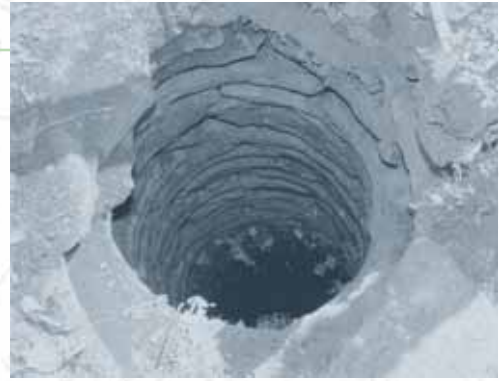
Built with generally flat stones, the walls of this well have also been cut to match the curve of the wall.
