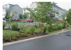
Stormwater infiltration / rain gardens
