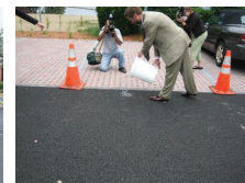
Porous asphalt & permeable pavers
