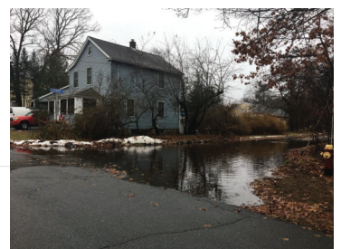
Photo: Pupkis Road Flooding
