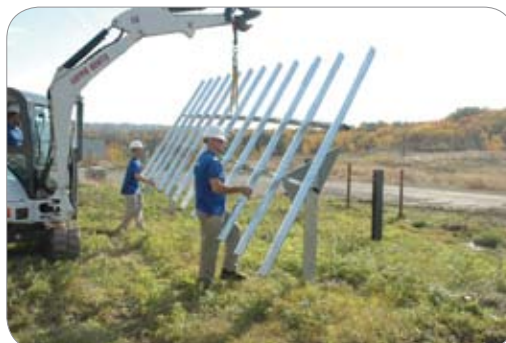
Figure 6: Driven Pile Mounting Structure (photo: Solar FlexRack)
