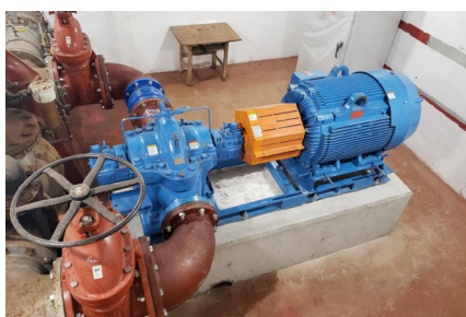
10 kW pump as turbine installed at the Narrows Road Water Treatment Plant in Fitchburg, Massachusetts
