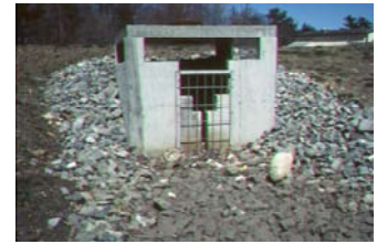
Outlet structure for detaining a range of flows
