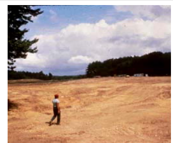
Dry dredging: removal to “hard” bottom (provided by C. Carranza of BEC)
