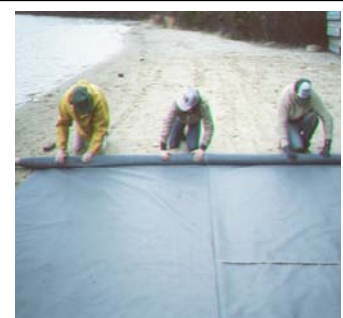
Preparing benthic barrier for easier installation
