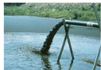
Hydraulically dredged slurry deposition
