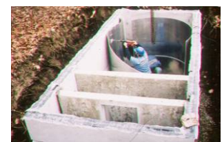
Advanced grease and grit trap (Vortech)
