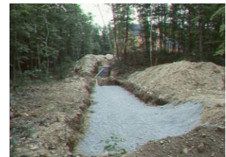
Septic system leachfield being installed
