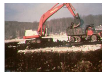
Dry dredging with conventional excavation equipment (provided by C. Carranza of BEC)
