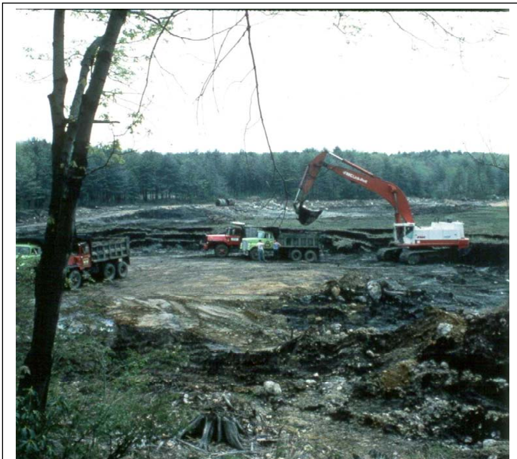
Dry dredging: excavation of dry lake bed (provided by C. Carranza of BEC)
