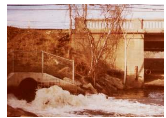
Drawdown pipe (left) usurps flow from normal outlet (right)
