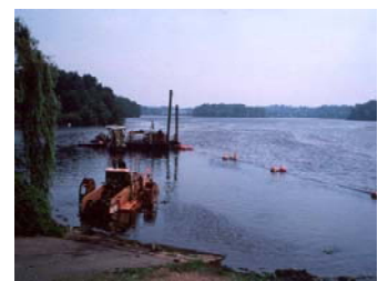
Hydraulic dredging: dredge in background with buoyed pipeline
