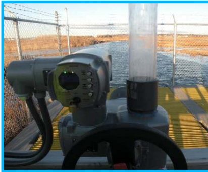
Electric Actuator with Manual Hand Wheel in Foreground
