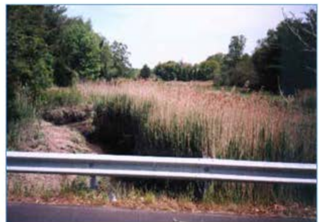
Photo of upstream impoundment dated 6/25/2015
