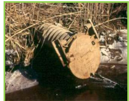
Top-Hinged Flapper Gate with no Control Mechanism
