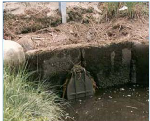
Photo of tide gate dated 6/25/2015
