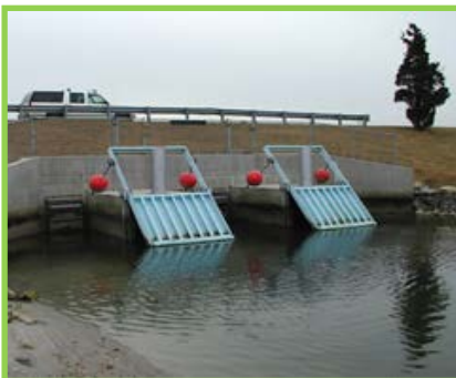
Self-Regulating Tide Gate with Counterweights
