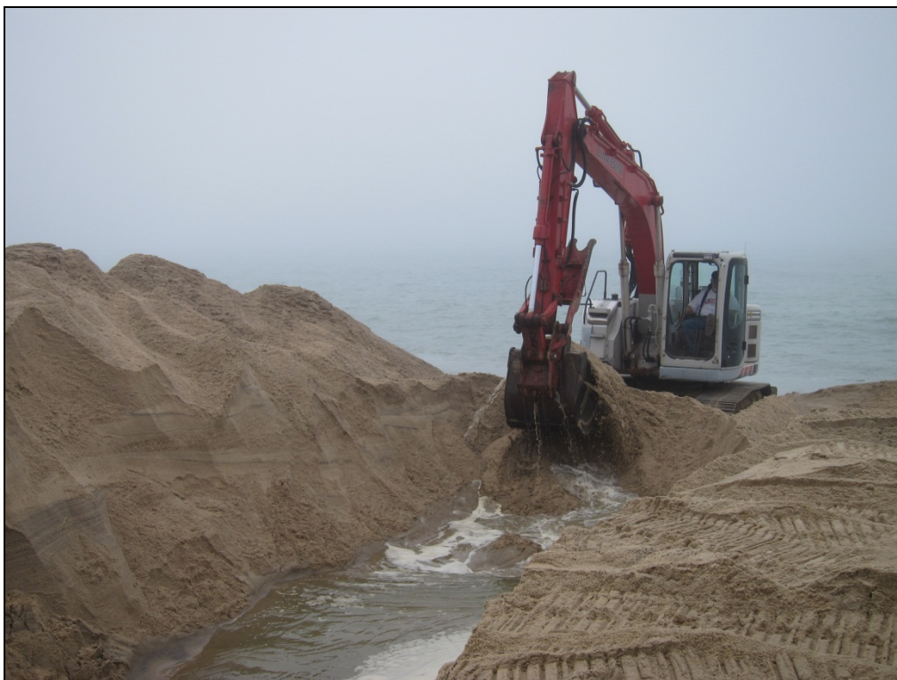
Figure V-2. Great Pond inlet excavation by a backhoe, March 21, 2012.
