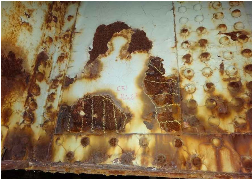
Heavy Corrosion in Lower Web and Flanges - Steel Cross Girder
