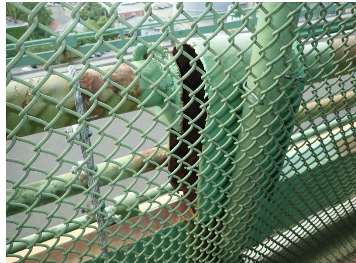
Disconnected Top Rail
