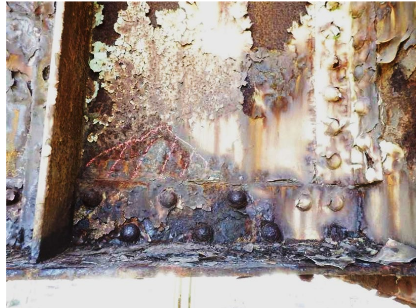
Close up of peeling paint
