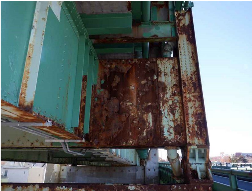
Lower Level Paint Condition
