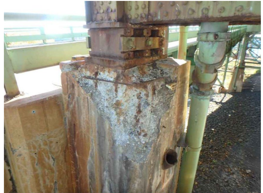
Spalling of Concrete at Pier Column with Exposed, Corroding Reinforcing
