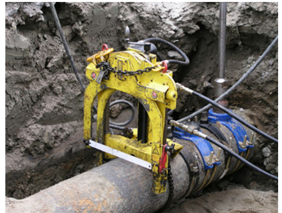
When possible, select tools that don't have potential for kick-back. This hydraulic cutter and diamond wire guillotine pipe cutter avoid kick-back forces.
