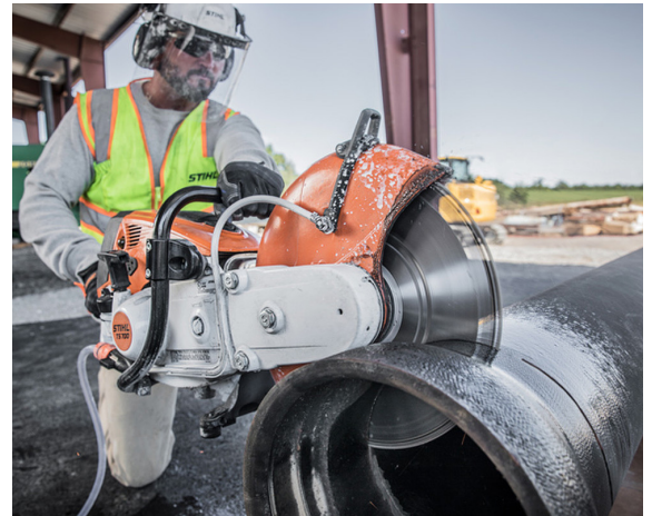
Circular blades can kick-back. Use the proper cutting area and make sure machine guards are in place.
