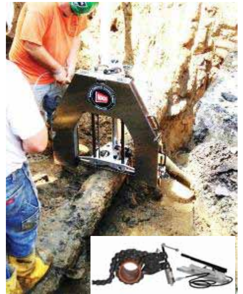
When possible, select tools that don't have potential for kick-back. This hydraulic cutter and diamond wire guillotine pipe cutter avoid kick-back forces.
