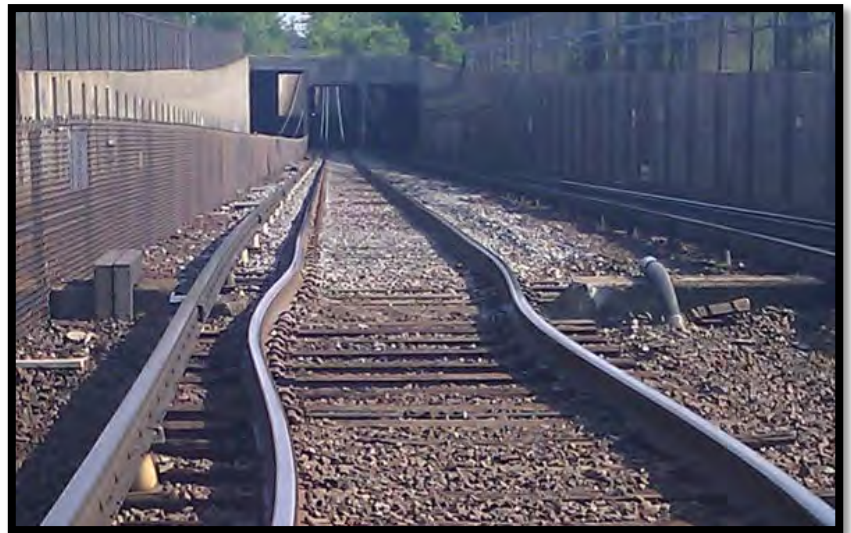
Figure 33 Heat kink on the MBTA Orange Line.
