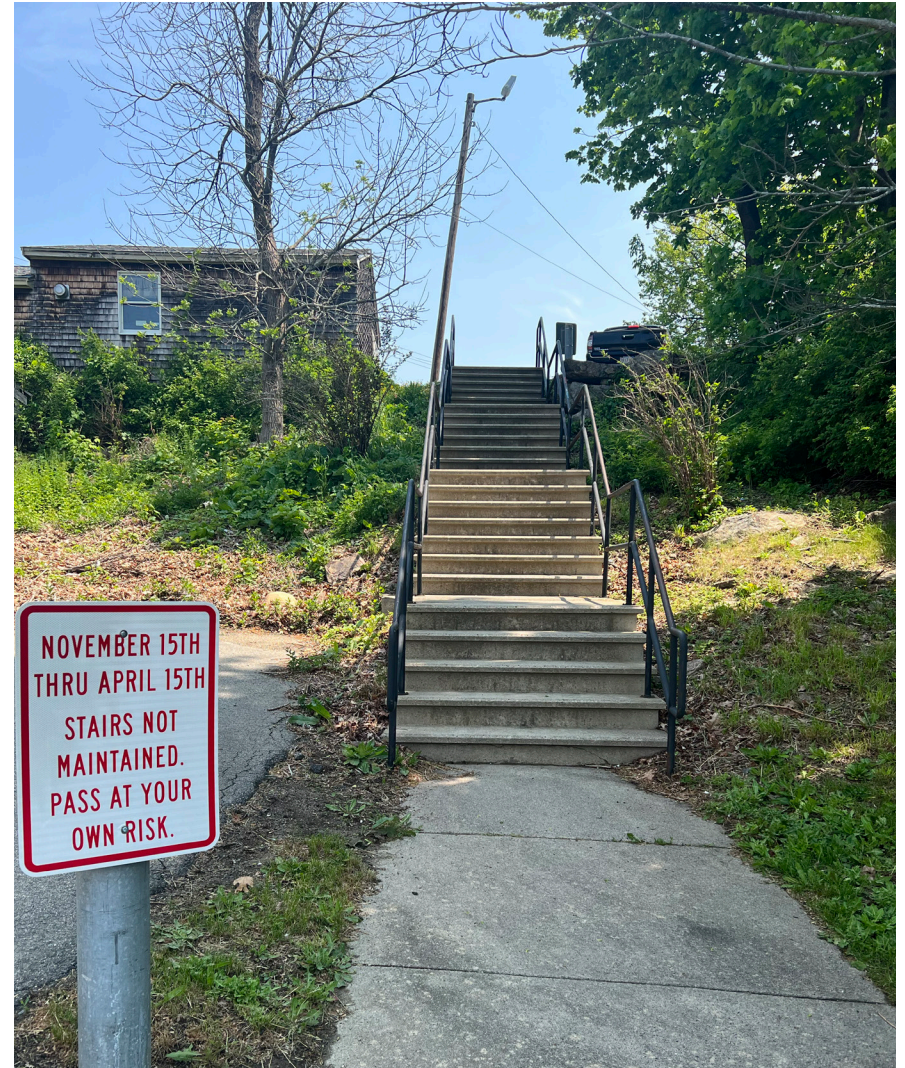
Staircase connecting the public parking lot to Main Street, which presents an opportunity to improve wayfinding cues for pedestrians.
