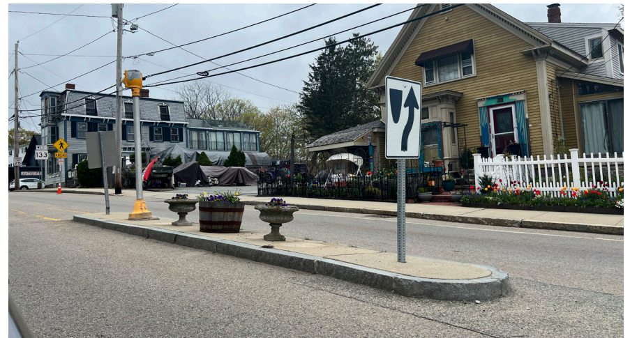
Existing planters on Main Street near the Martin Street intersection.
