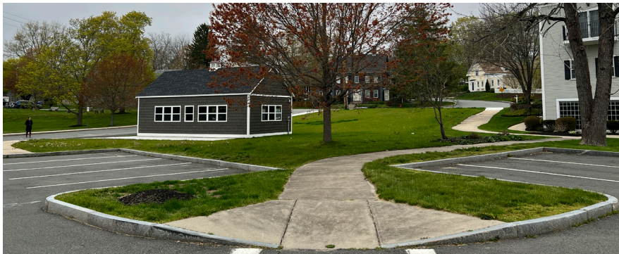
View of 24 Martin Street from the public parking lot.
