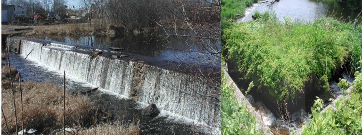
Figure 2: The Acushnet Sawmill Dam (left) and original weir-pool fish ladder (right) prior to construction in 2007.
