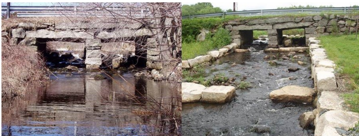
Figure 9: Completed construction (October 2007) of the rock weirs downstream of Hamilton Street.
