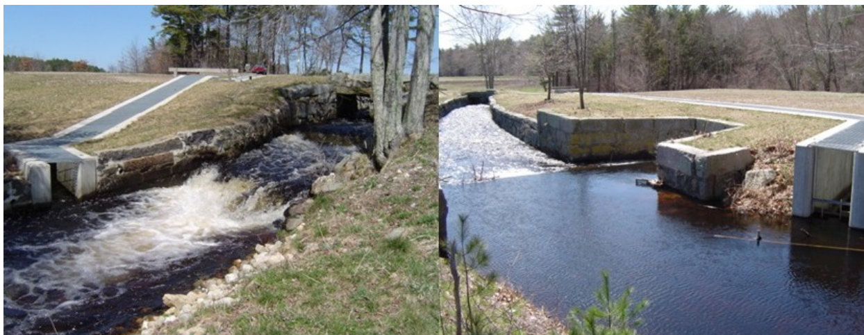
Figure 6: Downstream section of the New Bedford Reservoir showing the location of the Denil ladder entrance (left) and exit upstream (right).
