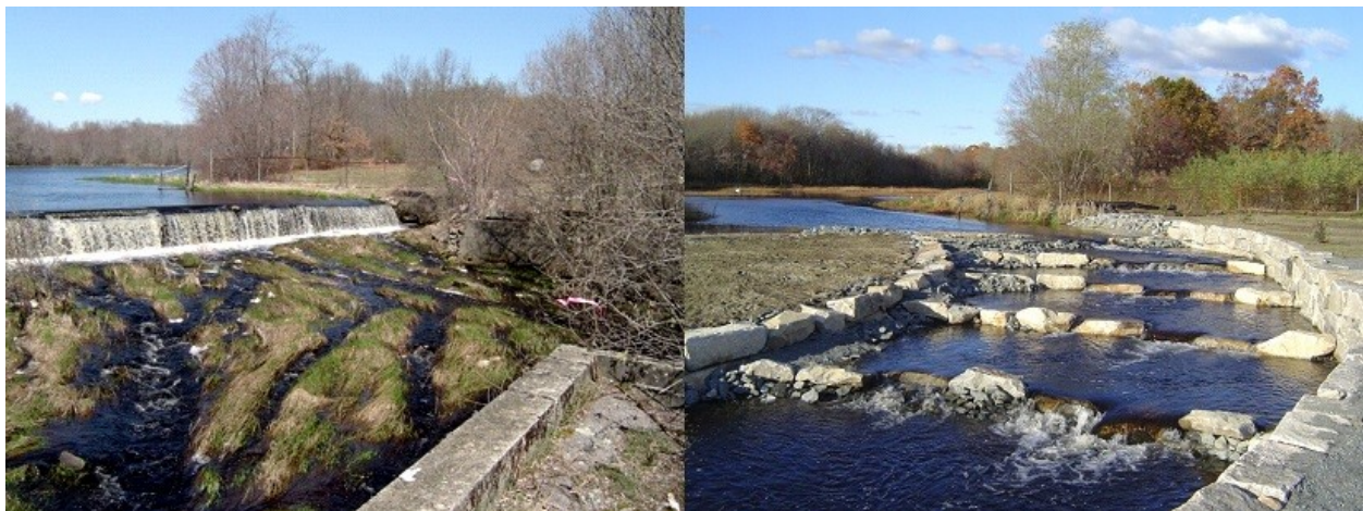
Figure 8: The Acushnet Sawmill dam and fishway prior to (April 2007, left ), and after (July 2007, right ) construction.
