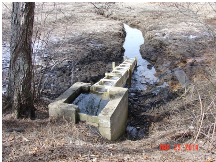
Figure 4. New Tom Matthews Pond fish ladder constructed in March 2014.
