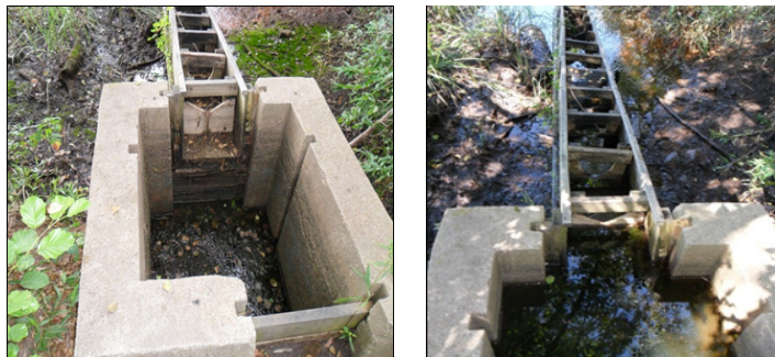
Figure 3. Concrete box and Denil fish ladder in 2012. Note the difference in the box water level between July (left) and October (right).
