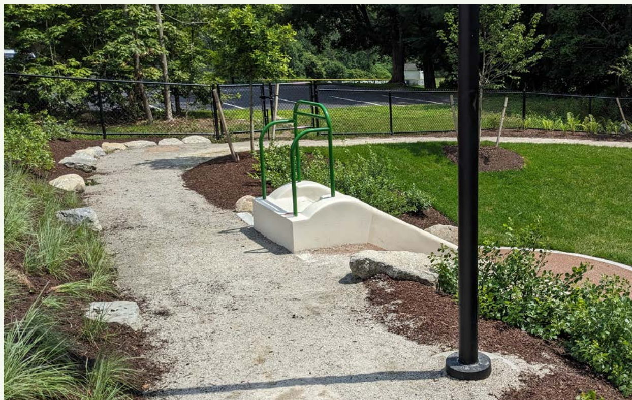
Stabilized Crushed Stone at Upton Community Center
