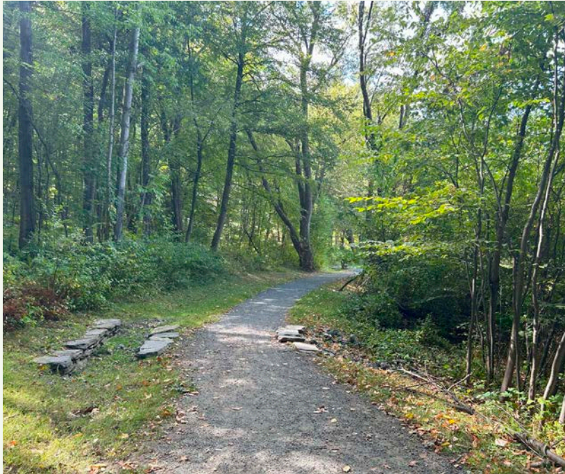
Left: Example of a trail at Mount Tom North Trailhead Park in Easthampton, with a crowned surface that pitches water to each side. The uphill side is graded into a swale, with a basin and culvert at intervals to carry water underneath the trail to a downhill outfall. Maintaining a low turf edge allows water to sheet off the side of the trail, avoiding any flow down the length of the trail surface.
