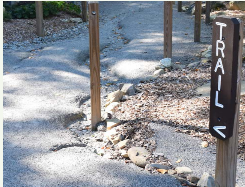
Above right: Example of water scouring on a trail. Above left: Example of sub-grade culvert and swale installed to prevent water running over the surface of the trail.
