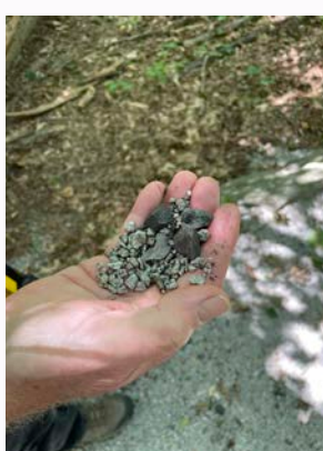
Surfacing patched with incorrect size aggregate
