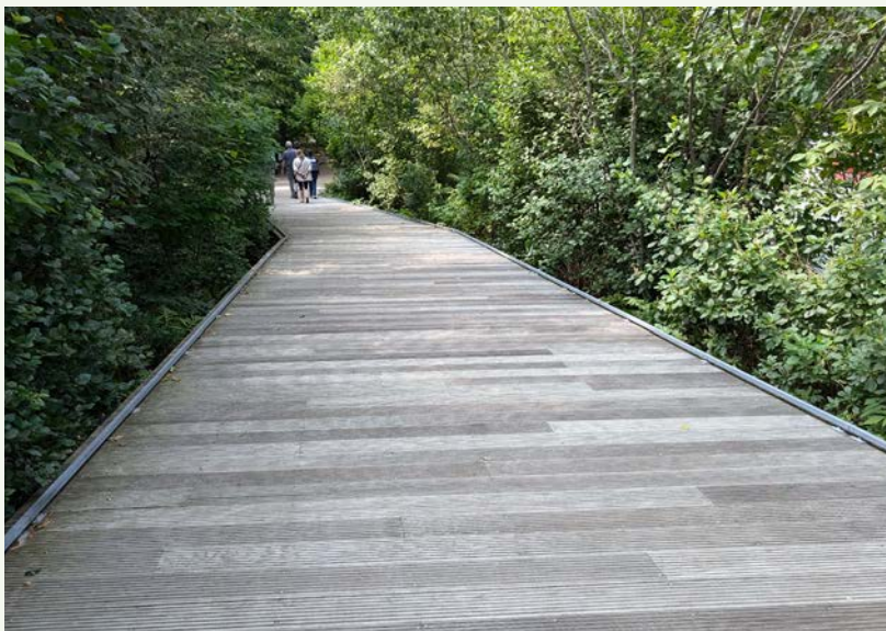
Thermally-modified hardwood boardwalk at Walden Pond
