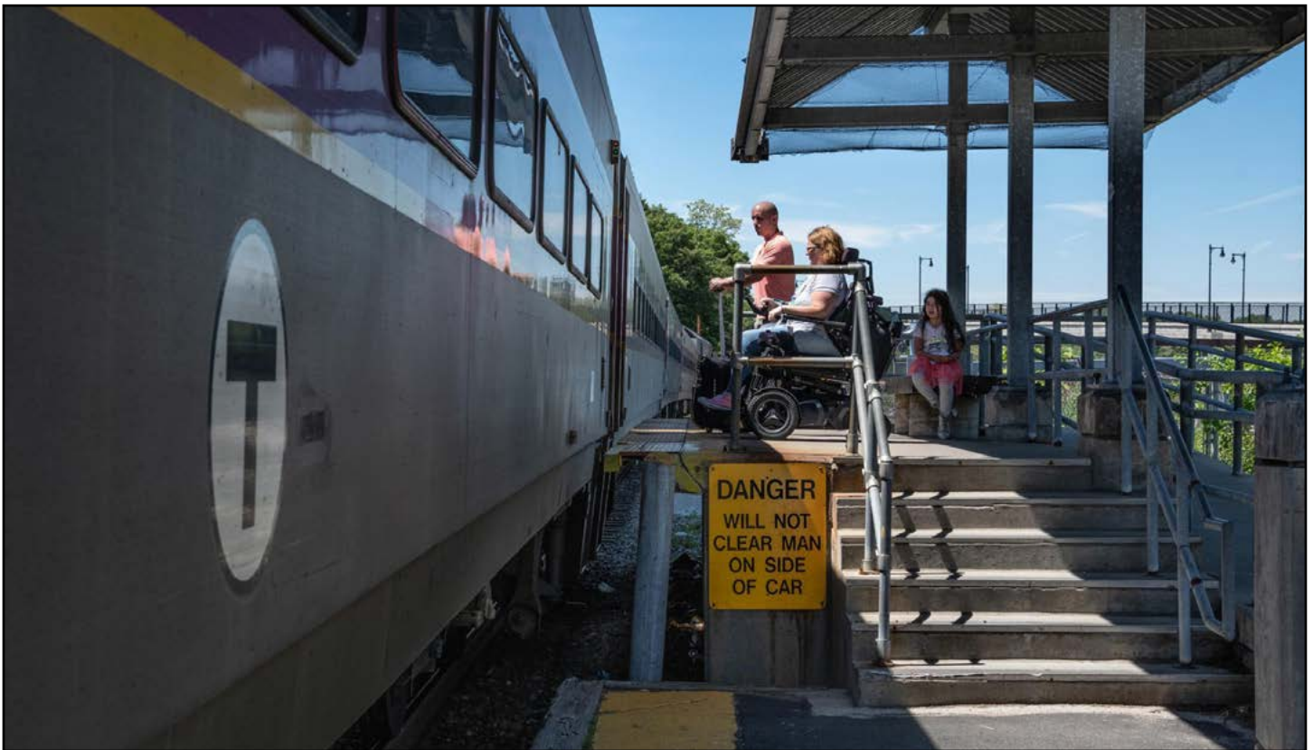
Pictured Above: Example of a mini-high platform at an MBTA Commuter Rail Station.
