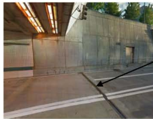
Photo 8. Typical Portal Drain
