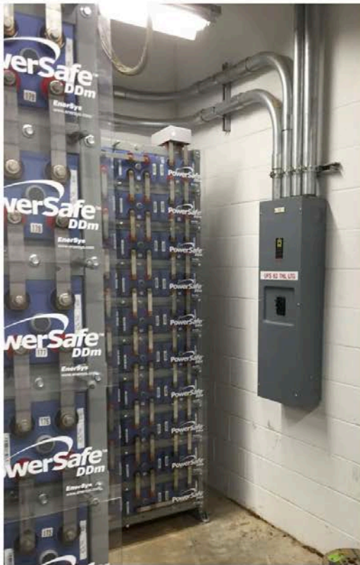
Photo 5.0 – UPS Batteries in Basement
