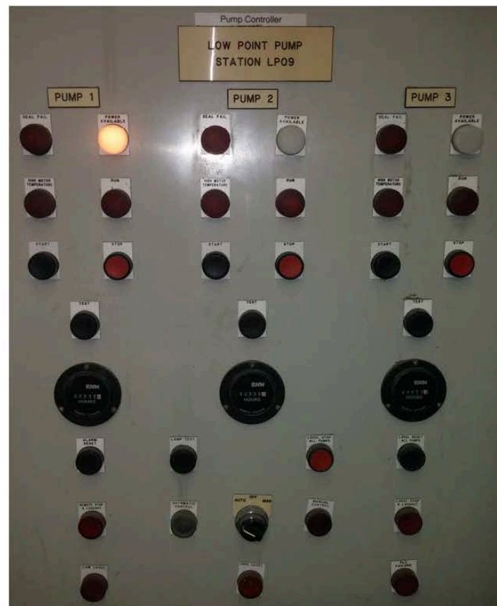
Photo 15. LP09 Pump Controller (LP08 similar)
