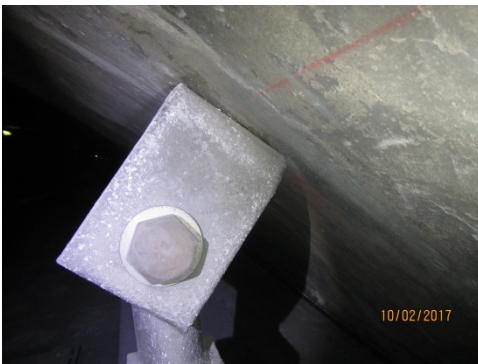
Liner Imperfection: bulge not attributed to failure (i.e. imbedded utility)
