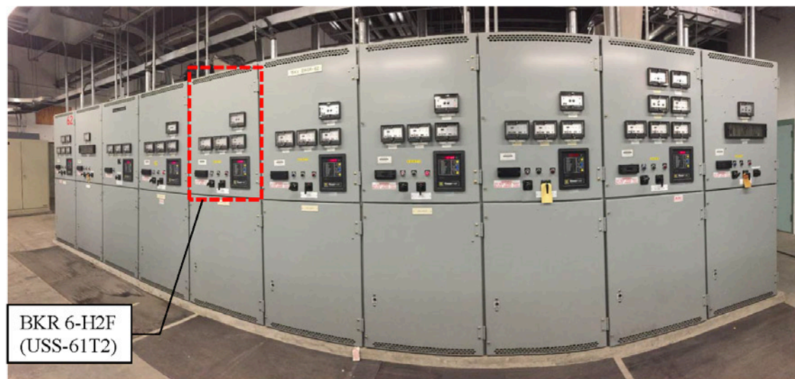
Photo 1.0 – Panoramic View of VB-6 Switch Gear No.2 (SWGR-62)
