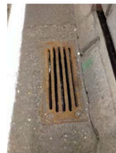
Photo 3. Roadway Drain Inlet Box
