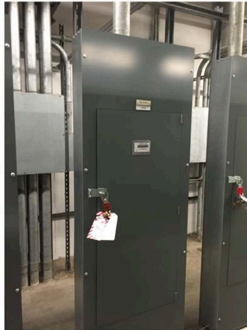
Photo 9.0 – LTG Panel with Lockout/Tagout
