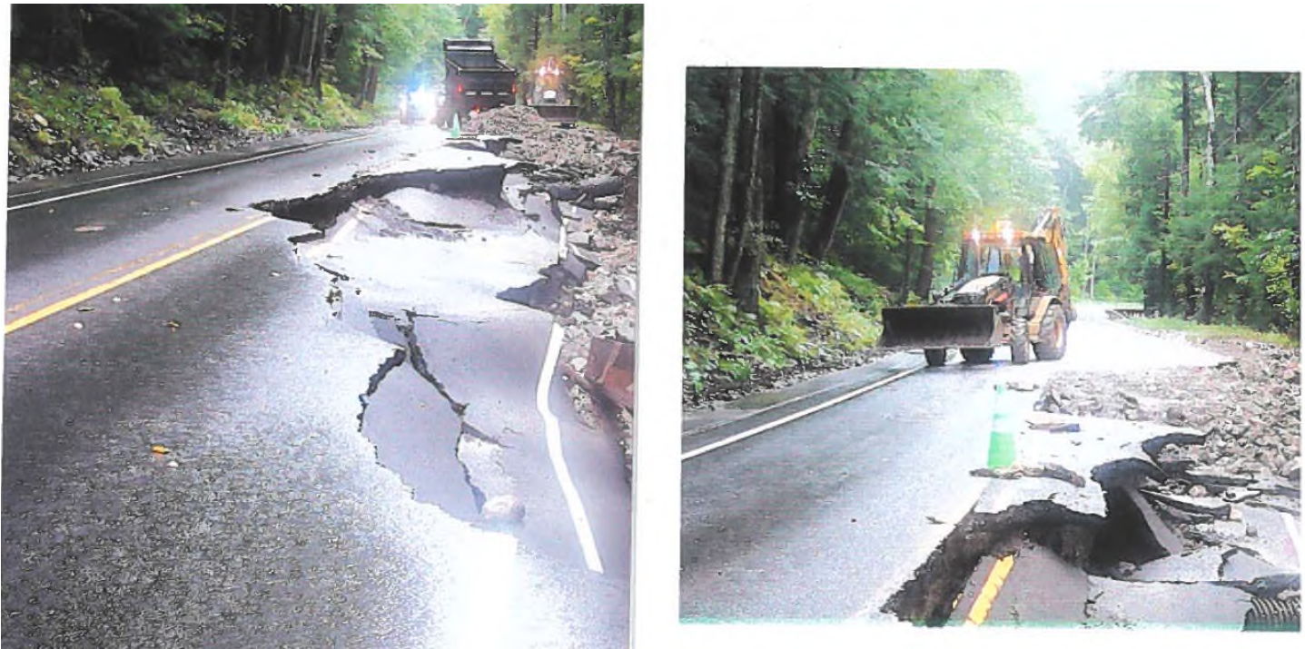
Figure 4. Damage to Main Road as a result of beaver dam breach in 2012
