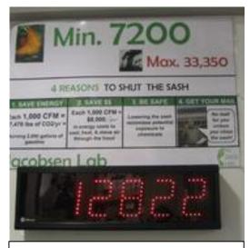
Simple displays and directions to show exhaust air flow rates and users' impact in fume hood driven spaces. The graphic above is from Harvard University's Jacobsen Lab.
