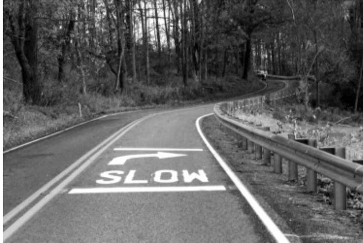
**Figure 10. Slow-down pavement markings on two-lane rural highways in Pennsylvania**
