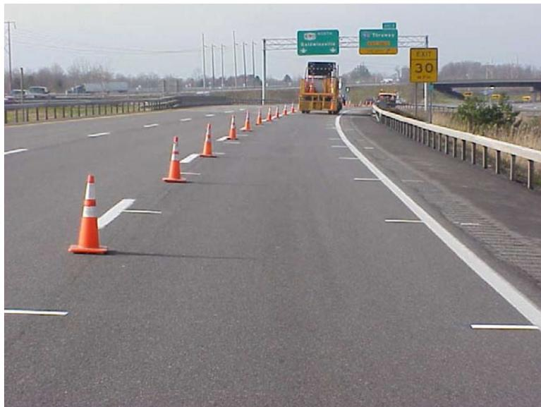
**Figure 13. Peripheral transverse pavement marking treatment on I-690 in Syracuse, New York**
