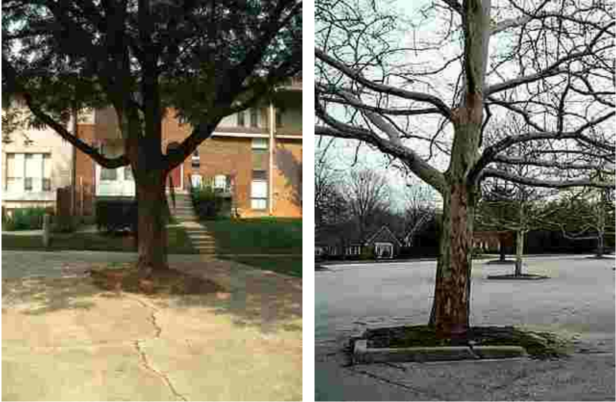
Figure 39. Trees planted in holes that are too small may eventually crack nearby pavement.
