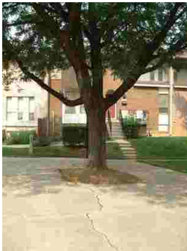
Figure 16. Tree roots cause adjacent pavement to crack.
