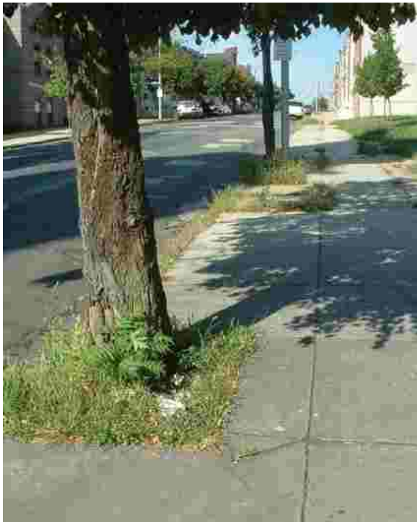
Figure 5. Typical urban tree pits provide only about 50 cubic feet of soil.
