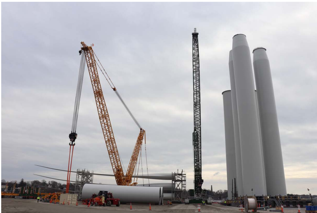
Figure 8. Tower components for the South Fork Wind project await transportation at State Pier in New London, Connecticut. Photo from Matilda Kreider, NREL
