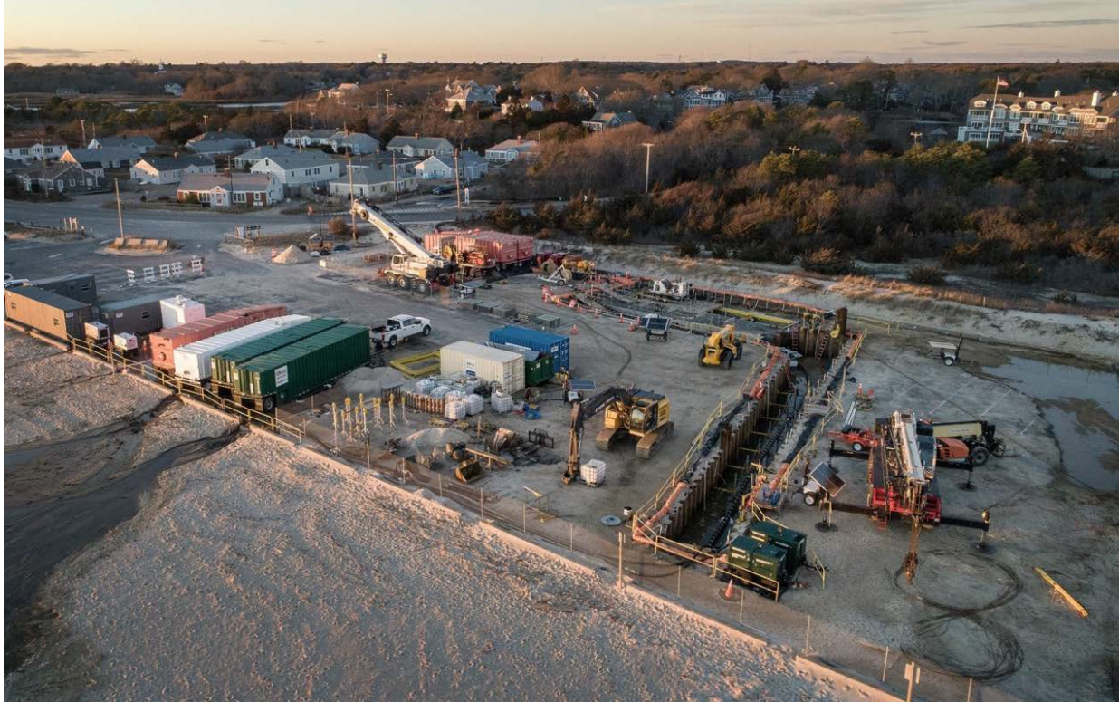
Figure 25. Construction occurs in the parking lot at Covell's Beach in Barnstable, Massachusetts, the location where cables from the Vineyard Wind 1 project come onshore. Following the completion of construction, this trench was covered, leaving no lasting visual impact or impact on use of the area. Photo from Robin Lubbock, WBUR
