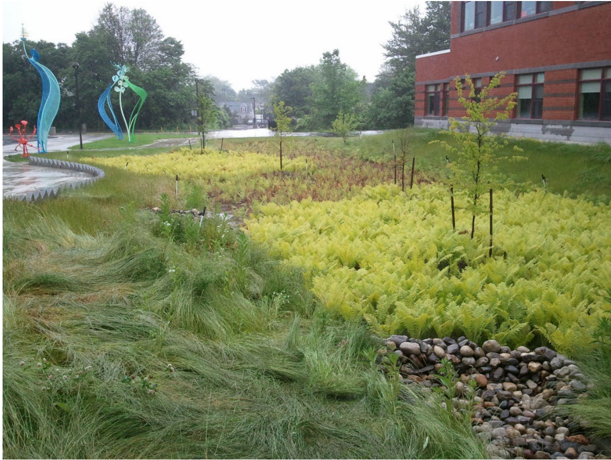
Figure 3.9: Bioretention Cell (City of Portland, n.d.)
