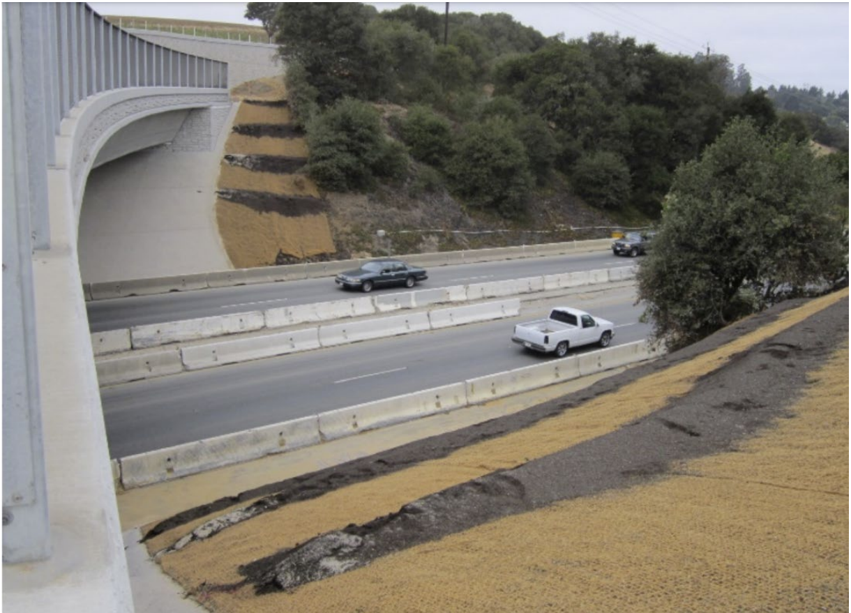
Figure 3.13: Compost Berm
