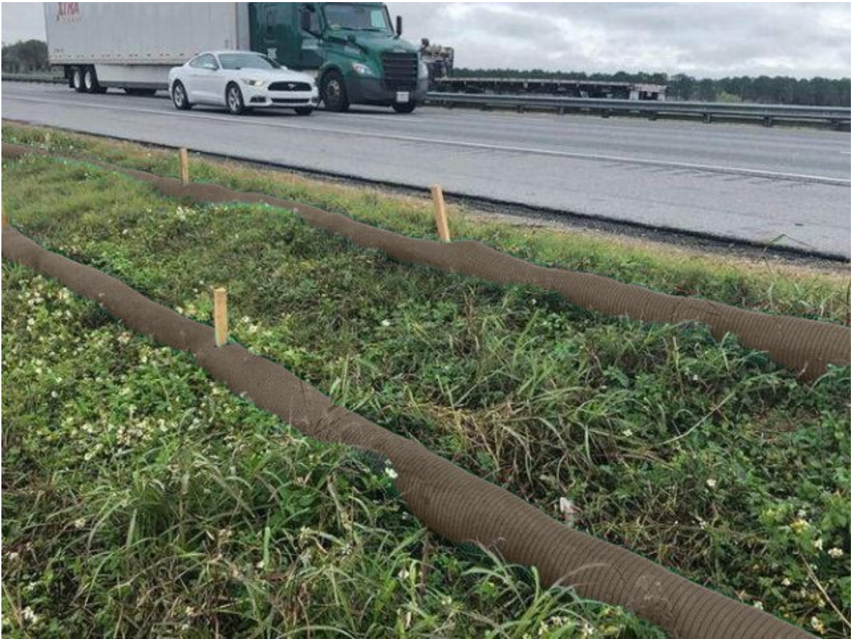
Figure 3.11: Compost Filter Tube
