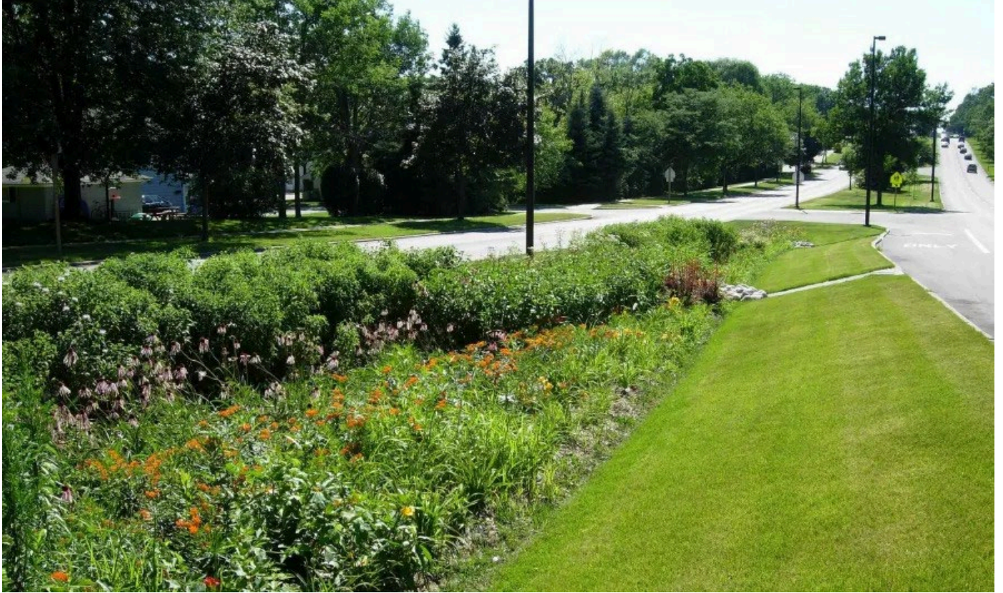
Figure 3.16: Bioretention Cell with Woodchip Overlay
