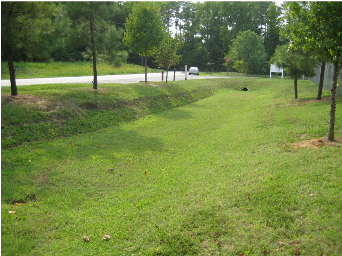
Figure 3.15: Bioretention Cell
