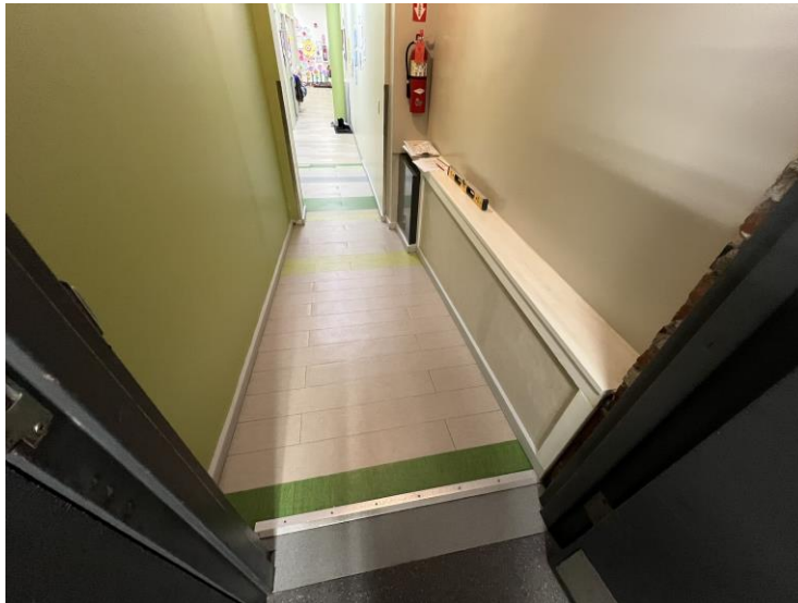
Figure 2: Existing Ramp Condition
