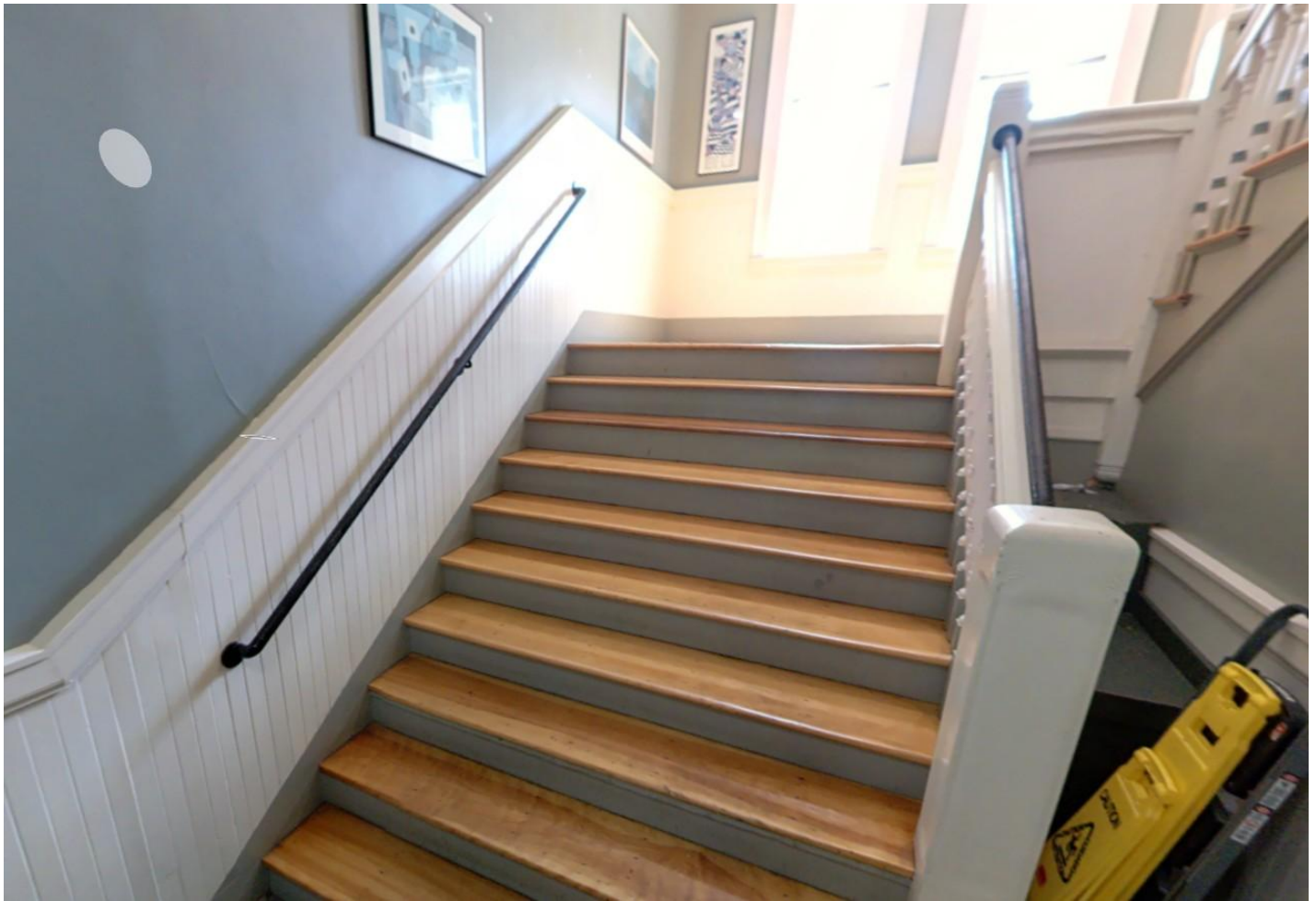
STAIR A - VARIANCE REQUEST 5 - 27.4.3 - HANDRAIL EXTENSIONS
