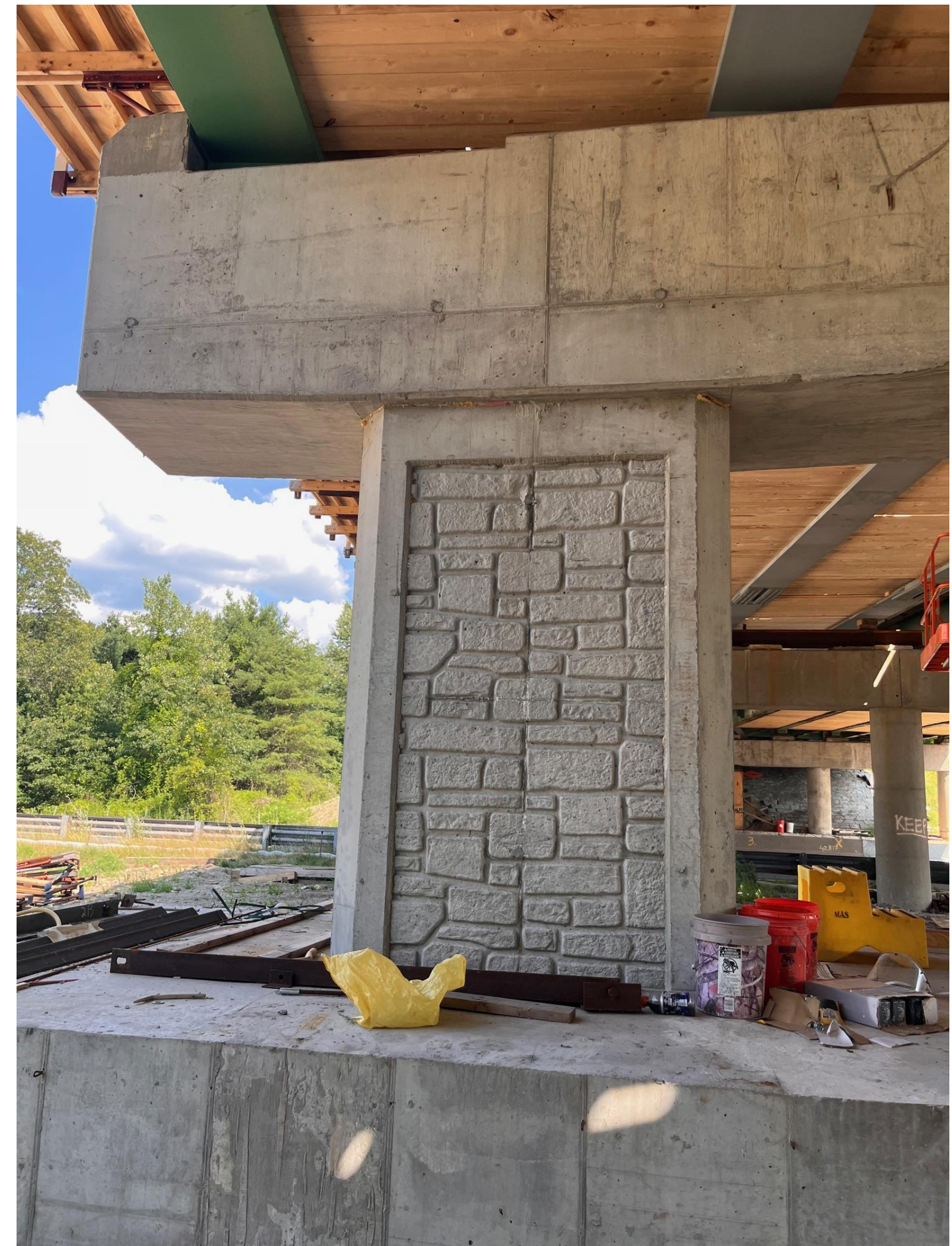
Current MassDOT aesthetic pier – Boxborough, Route 111 Bridge Replacement – July 2025
