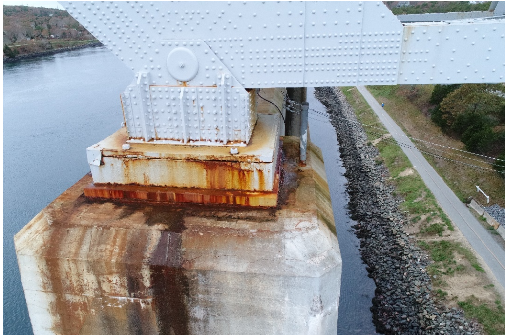
Figure 15: Image of bridge bearing, Massachusetts
