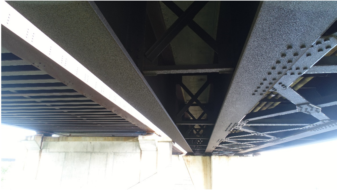
Figure 11: Underside image of a rail bridge deck to check for corrosion
