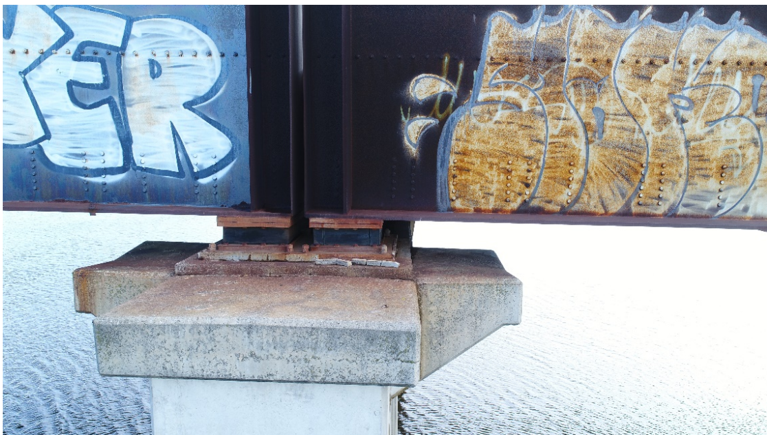
Figure 12: Image of deck bearings of the same rail bridge
