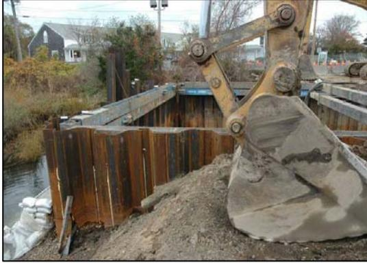
Construction work involves placement of sheet piling coffer dams to keep tidal flow out of the construction area, a temporary fish bypass culvert to allow herring to pass through, and installation of culvert, headwall and sidewalls.
