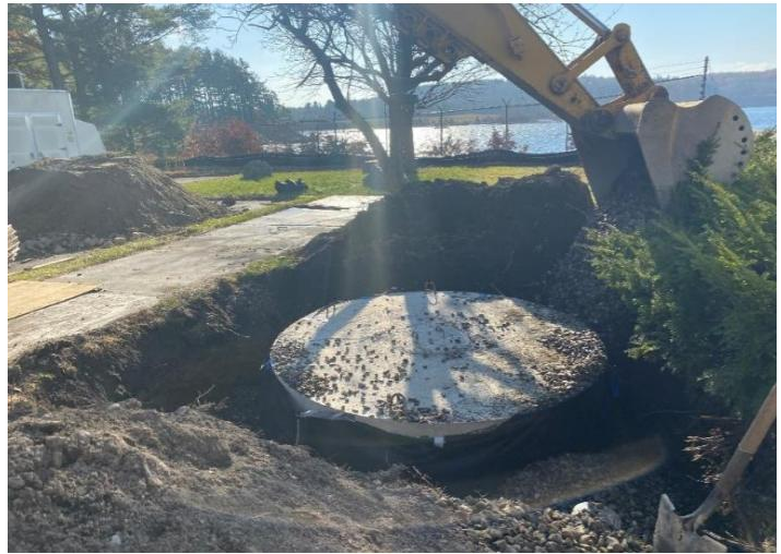
Drywell containing flow from deck drains
