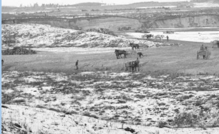
Covering muck on Section 8, east of Love's, Clinton; Sterling, Jan. 9, 1902
