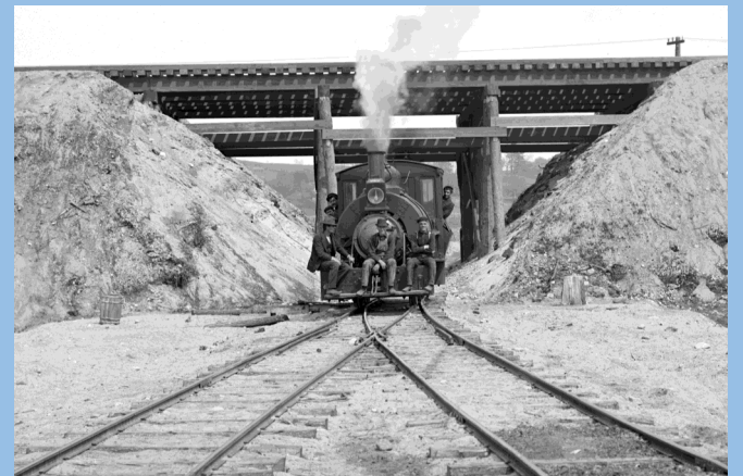
Sept. 29, 1905. Oakdale Quinapoxet River Channel. The river channels were widened and excavated. The hard soil and large boulders that were removed were used as embankments, berms along the Central Massachusetts Railroad above Oakdale, and for surfacing new roads.
