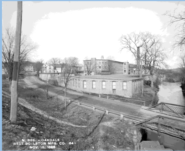
(Above) Nov 10, 1896. West Boylston Manufacturing Company from the Central Massachusetts Railroad tracks near bridge, Oakdale. The black stripe on the left telegraph pole indicates the future high water mark of Wachusett Reservoir. Everything below was removed or relocated.
