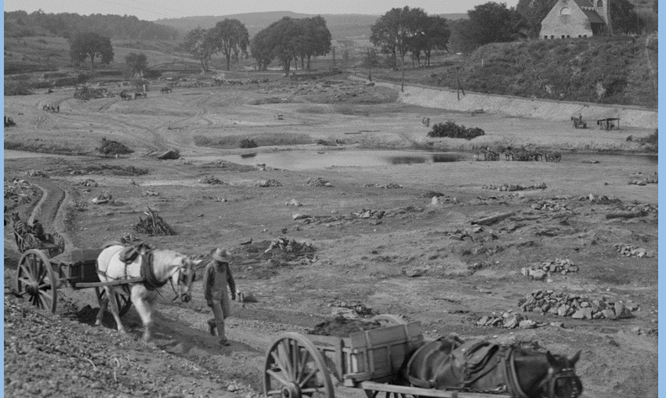
September, 1904. Stripping at the site of the Baptist Church, West Boylston. Today known as the Old Stone Church and Thomas Basin.
