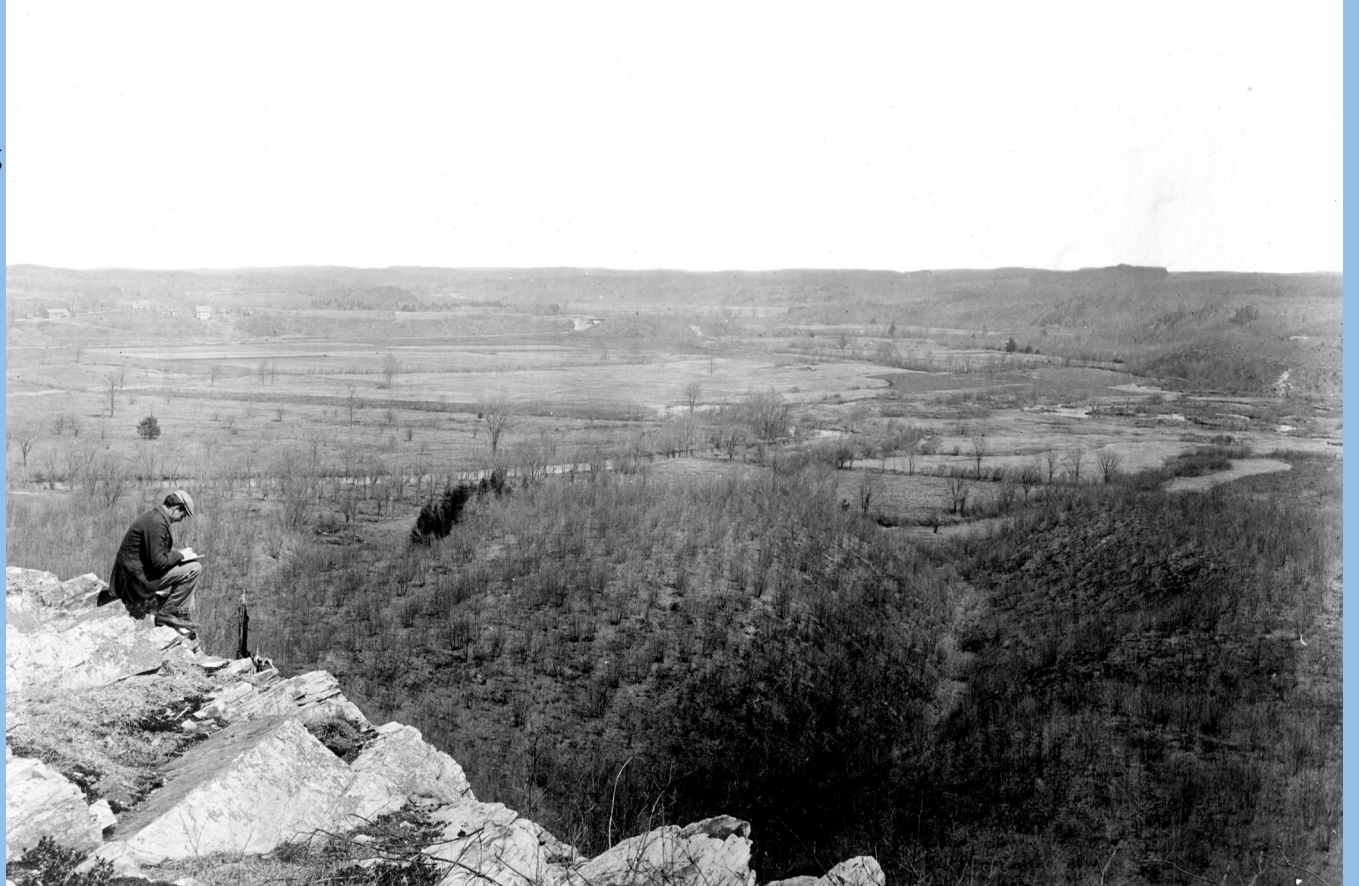
May, 1896. Site of "Nashua" Reservoir, before construction. Pine Hill, West Boylston.
