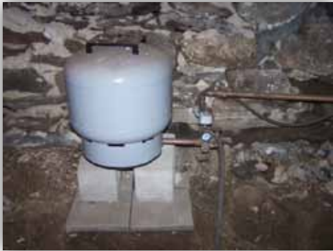
Storage Tank & Pressure Switch
