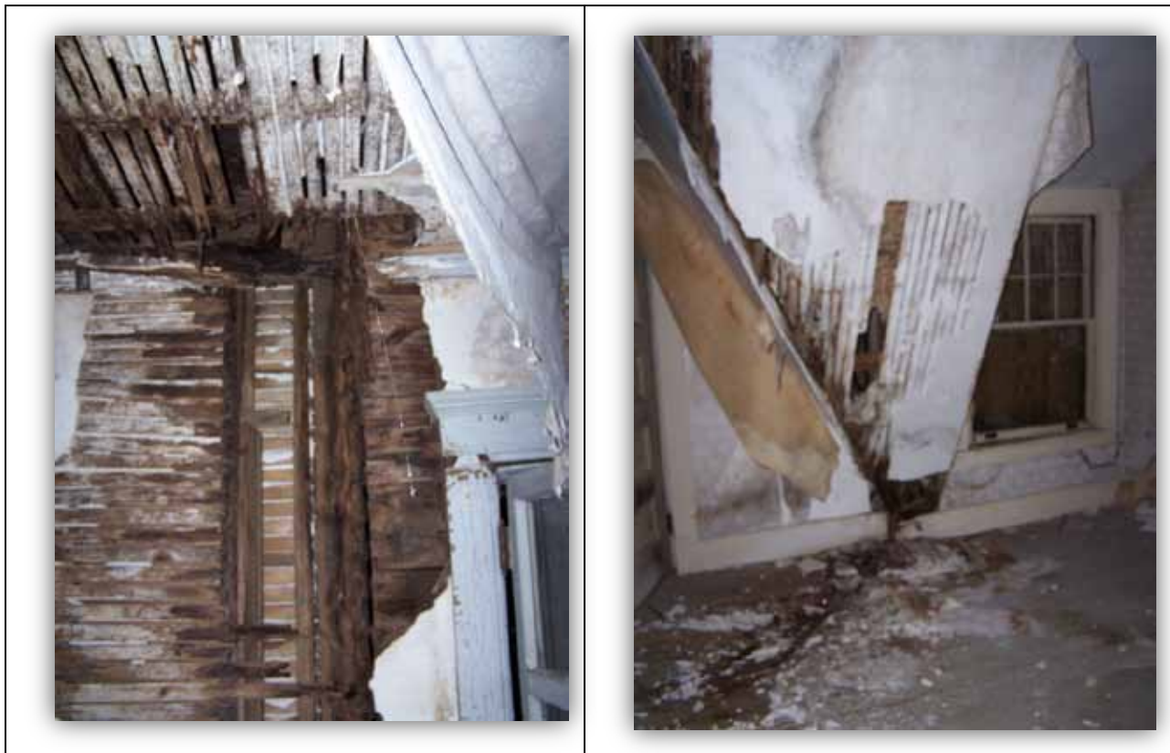
Water Damage @ Roof Level
