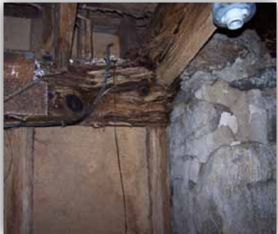
Failed Beam @ Sill
