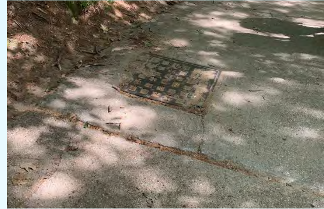
Sediment filled catch basin on E-ramp
