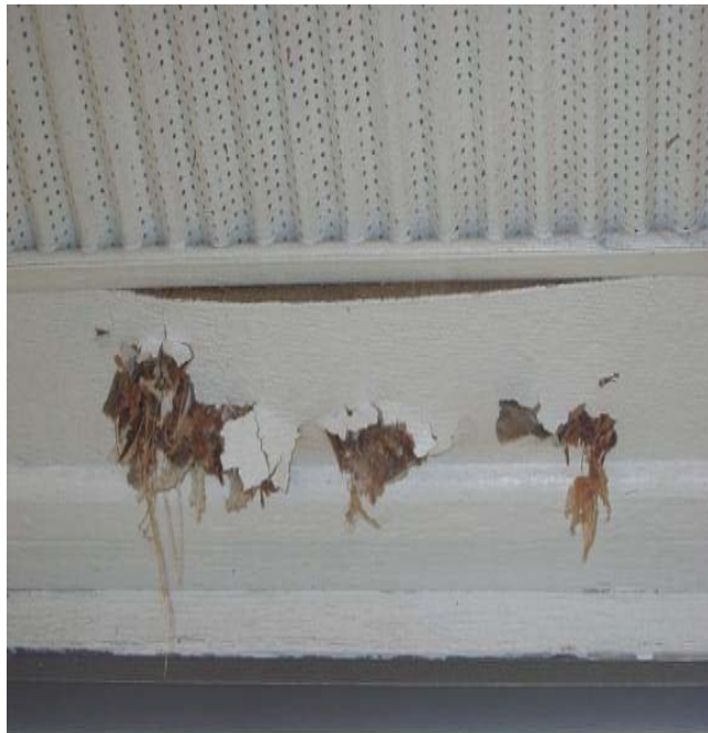
667-2 Development, Beaverbrook Apartments Beam above Walkway Is Rotting and Needs Replacement
