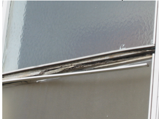
667-4 Development, 82 Orange Street Window in Common Area Needs Replacement
