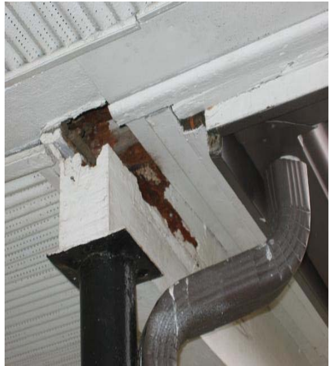
667-2 Development, Beaverbrook Apartments Portico above Sidewalk Is Rotting and Needs Replacement
