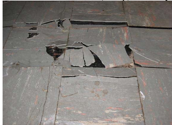
667-2 Development, 304 Grove Street, #3 Floor Tiles Are Broken, Damp, and Musty
