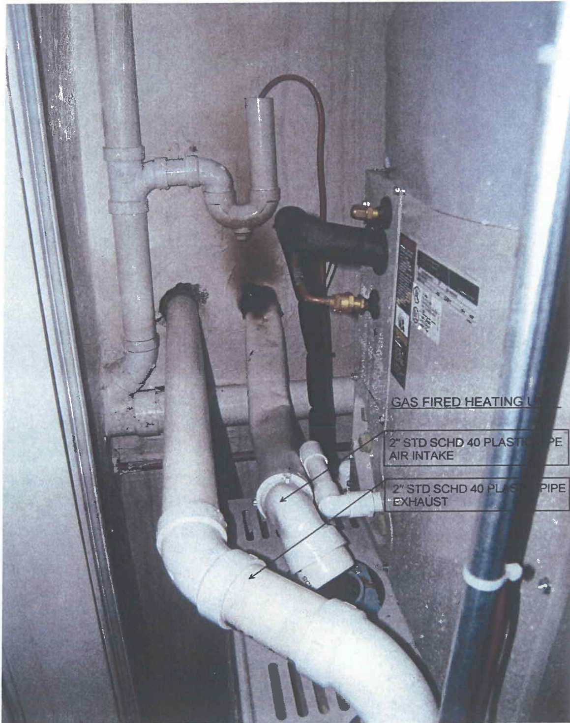
PHOTOGRAPH-NO. 7 - 47 Chestnut Street, Waltham, unit six - damaged plastic piping to gas fired furnace (Jan. 15, 2010)
