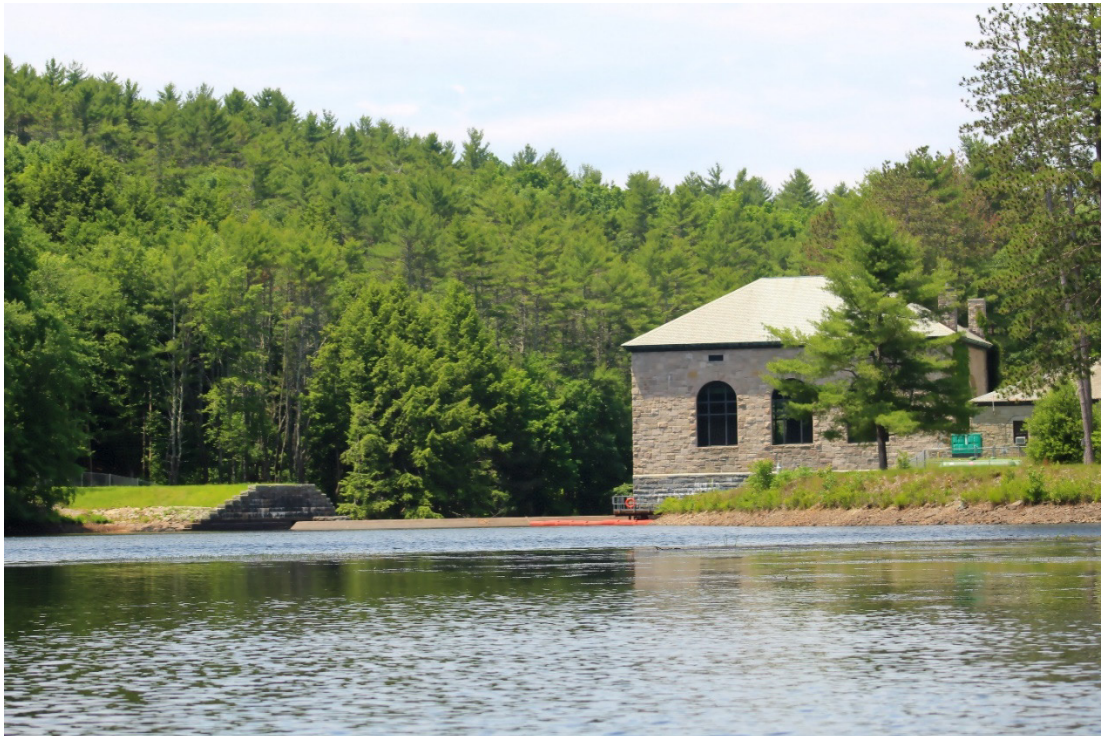
Ware River upstream of MWRA Shaft 8 horseshoe dam
