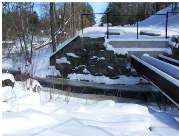
Rail trail abutments and new sewer lines in place awaiting bridge construction, 2009.
