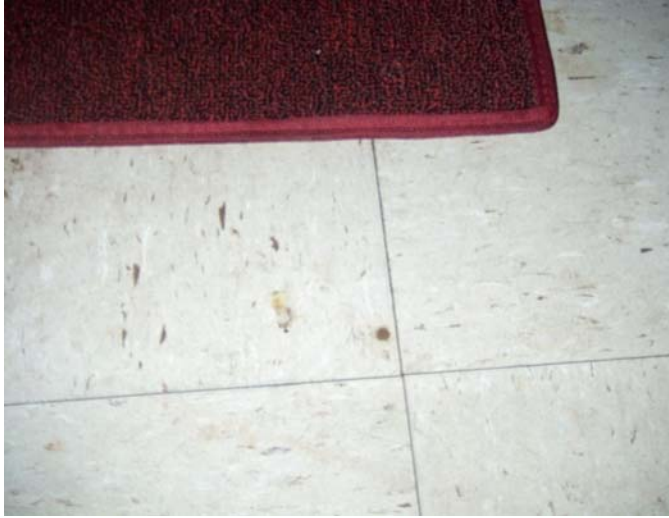
Project 667-1 Asbestos Tiles Nailed Down for Repair
