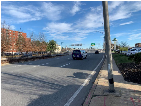
Figure 2.5-3: Sidewalk obstructions such as utility poles that obstruct the minimum four-foot-wide path of travel requirement for ADA accessibility - South side of Revere Beach Parkway.
