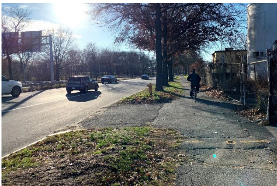
Figure 2.5-5: Poor pavement conditions making it difficult for people in wheelchairs or with strollers to navigate the sidewalk - North side of Mystic Valley Parkway
