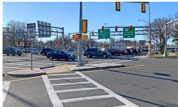
Figure 2.5-6: Crossing of several lanes of traffic and high vehicle speeds making an uncomfortable pedestrian environment even with marked crosswalks and paths - Wellington Circle
