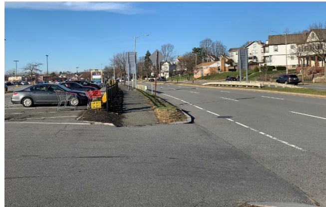
Figure 2.5-4: High frequency of driveways breaking up the sidewalk and creating conflicts between pedestrians and turning cars - West side of Fellsway north of Wellington Circle
