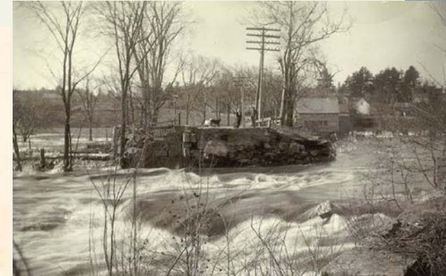
WB bridge destroyed by flood, 1900
