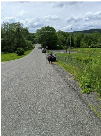
Figure 1: Looking toward the west over the pipe in the road.
