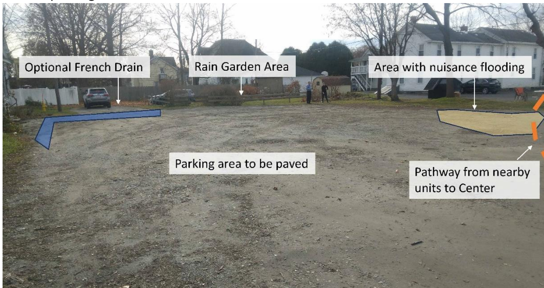
Photo C-33: View of proposed BMP locations with respect to the parking area
