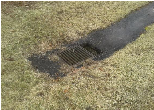
Photos 4 and 5: Asphalt swale leading to storm drain
