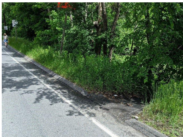
Photo C-3: Curb cut on Pecks Road
