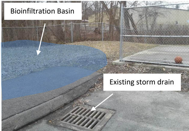
Photo C-41: Existing catch basin with Bioinfiltration basin
