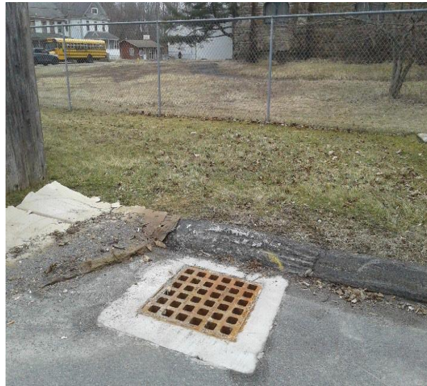
Photo C-44: Existing storm drain
