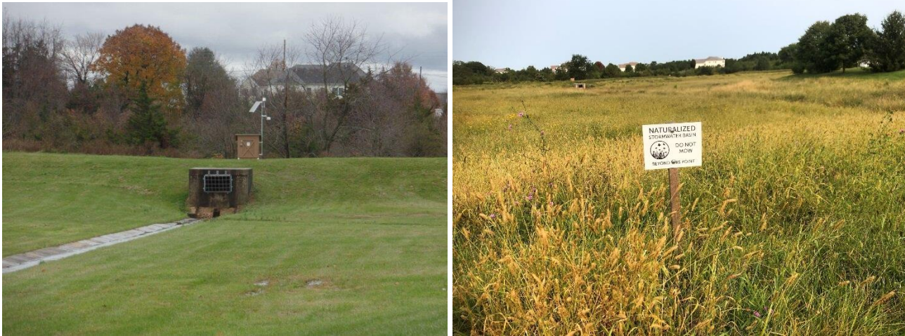
Photos C-48 and C-49: Pre- and Post photos of a retrofit stormwater basin at Laird Terrace, Franklin Township, New Jersey
