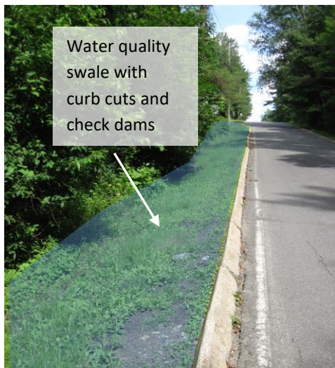
North side of spur road east of the curve.
