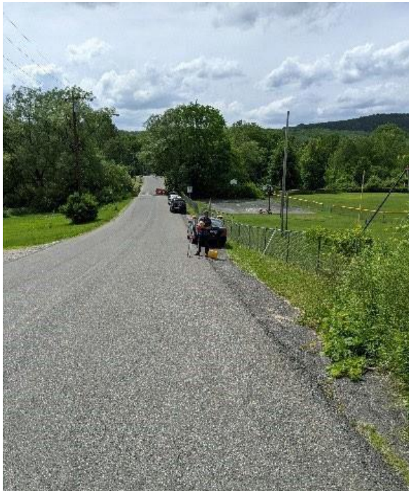
Photo C-13: Looking toward the west over the storm pipe in the road.
