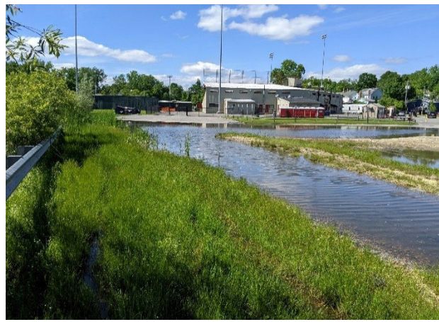
Figure 2: From the West, looking at the flooding in the parking lot.
