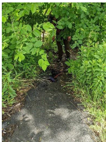
Photo C-4: Paved swale from curb cut draining directly into Onota Brook
