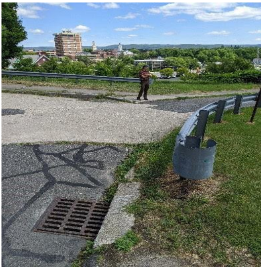
Photo C-5 (left): At the intersection with two shallow catch basins that drain toward 17 Francis Avenue
