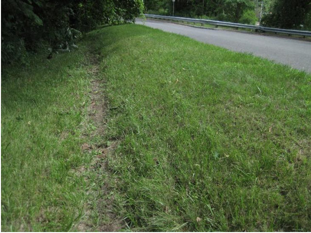
Photo 2: Existing swale with curbed parking area
