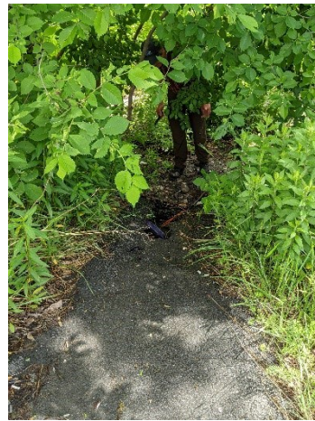
Figure 2: Paved swale from curb cut draining directly to Onota brook.
