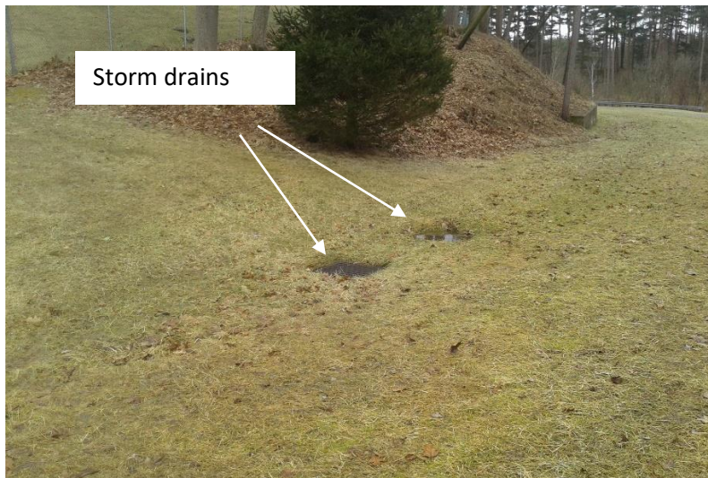
Photo 6: Storm drains located in existing lawn (1)
