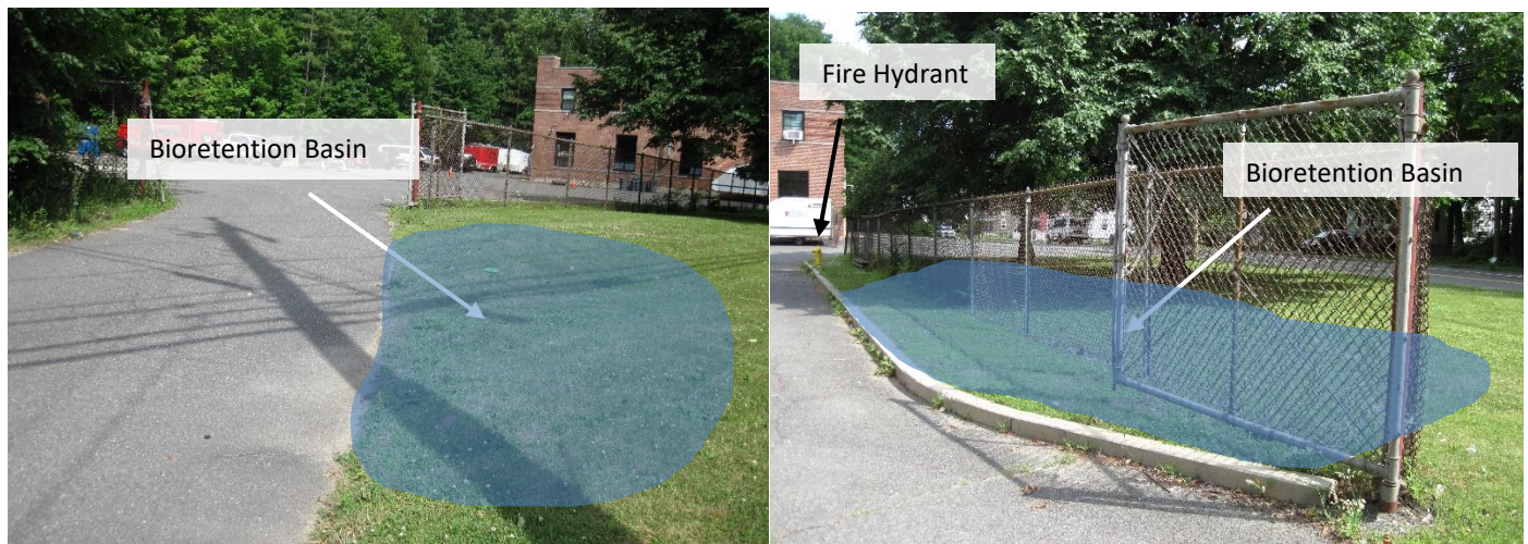
Photo C-32: Fire House entrance with Bioinfiltration basins locations
