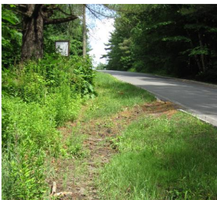
Photo C-30: An existing curb cut allows stormwater to enter the grassed edge. (North side of the access road east of the curve.)
