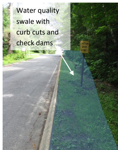
North side of spur road east of the curve.
