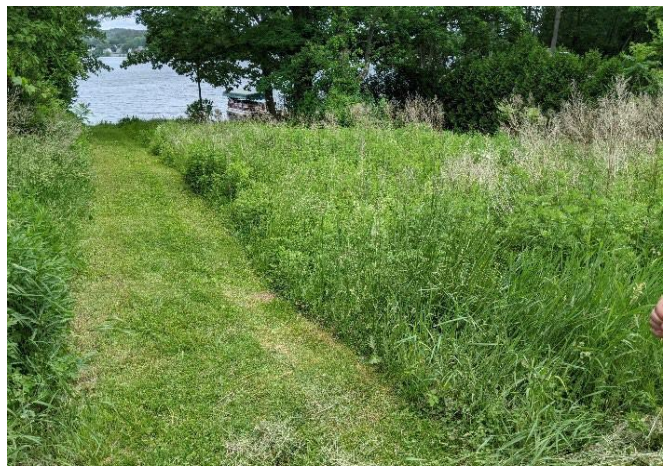
Photo C-12: Town easement sloped toward the lake - the location of the proposed bioinfiltration basin.
