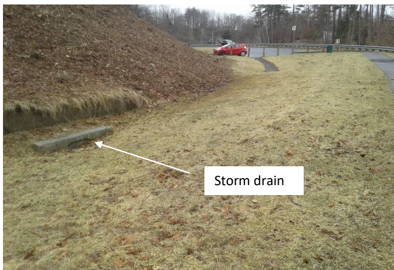
Photo 7: Storm drains located in existing lawn (2)
