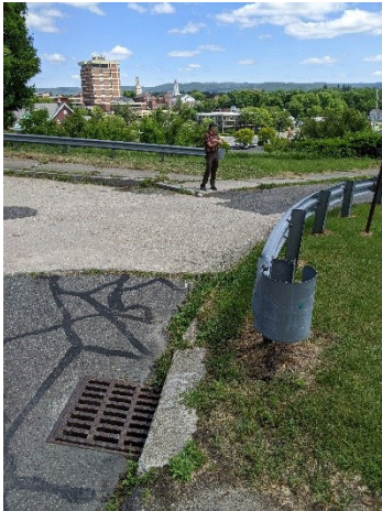
Figure 1: At the intersection with two shallow catch basins that drain toward 17 Francis Ave.
