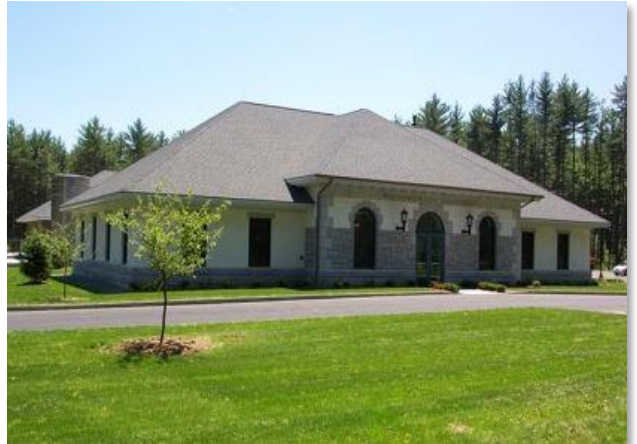
FIGURE 10: Forge Village Water Treatment Plant
