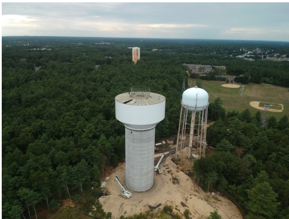
Figure 1-13 1.5 MG Coated Steel CET Under Construction (Middleborough, MA)
