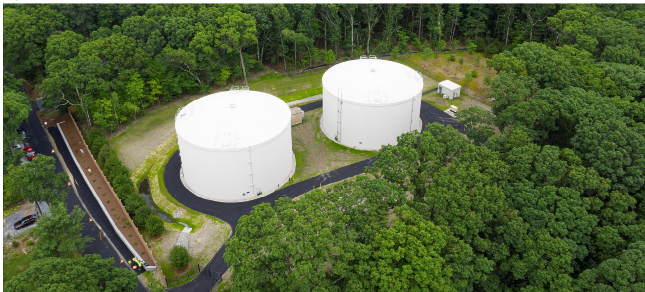
Figure 1-11 1.75 MG Prestressed Concrete Water Storage Tanks (Framingham, MA)
