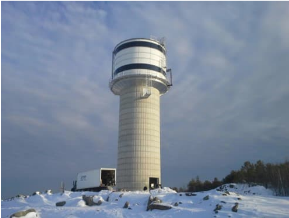
Figure 1-14 Glass-Fused-to-Steel Composite Elevated Water Storage Tank (Peabody, MA)
