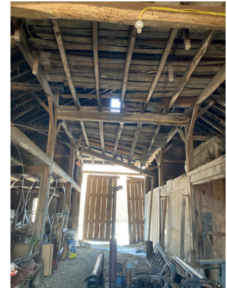
Wood post-and-beam framing is mostly sound and will require minimal restoration.
