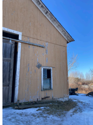
The main barn door facing North does not close fully and the window glazing is broken (left).
