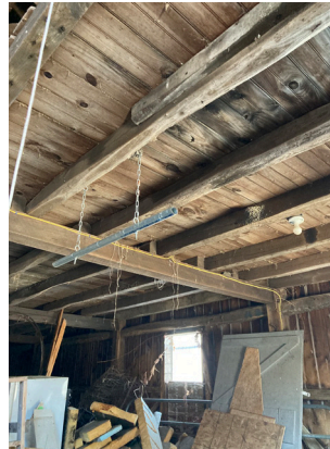
Wood post-and-beam framing is mostly sound and will require minimal restoration.
