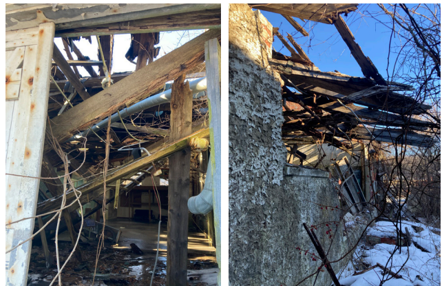
Looking through the front door (left) and along the side of the building (right), it is clear that the roof and wall framing are compromised and beyond repair.
