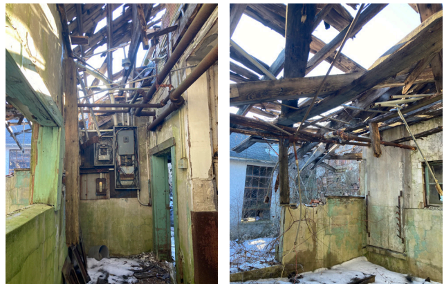
Looking through the front door (left) and along the side of the building (right), it is clear that the roof and wall framing are compromised and beyond repair.
