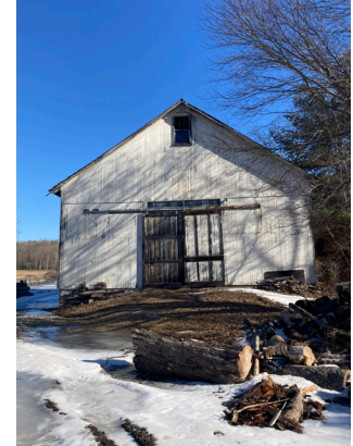
The main barn door facing North does not close fully and the window glazing is broken (left).
