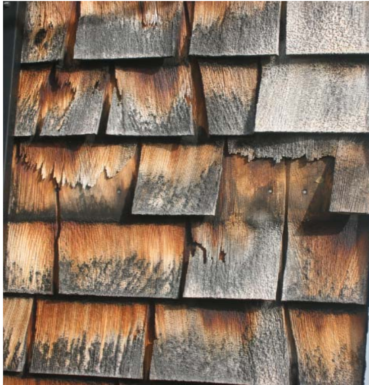
667-1 Development, 4F Greenwood Terrace Warped Shingles Need Replacing
