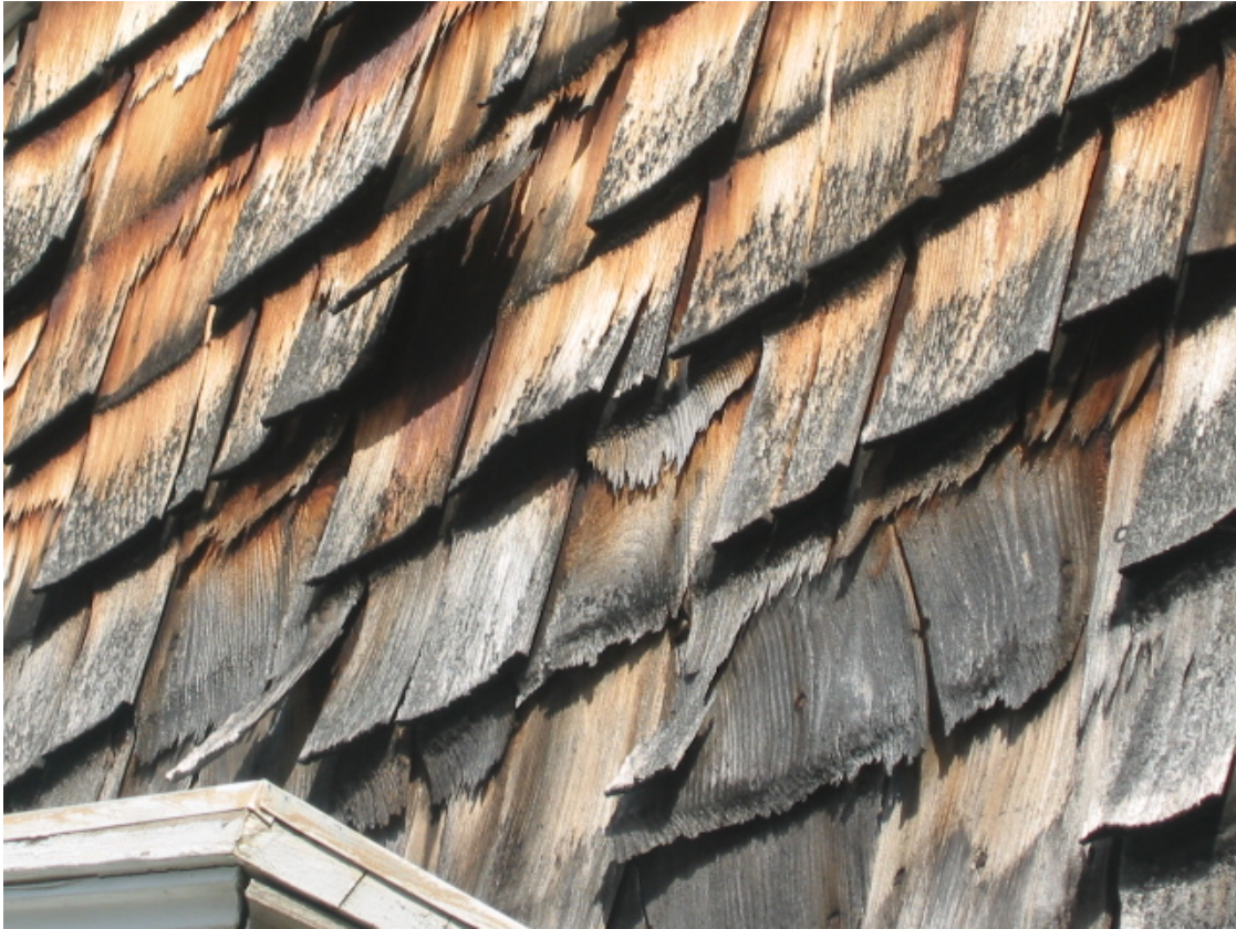
667-1 Development, 6A Greenwood Terrace Warped Shingles Need Replacing
