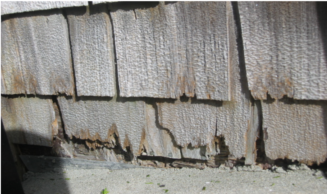
667-1 Development, 4F Greenwood Terrace Warped Shingles Need Replacing
