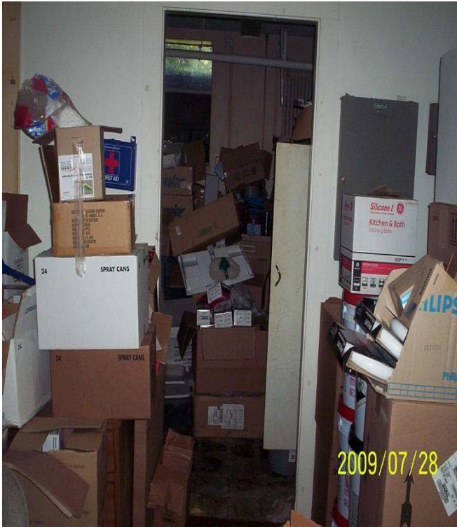
402 Essex St., 2nd Floor – Fire Hazard
